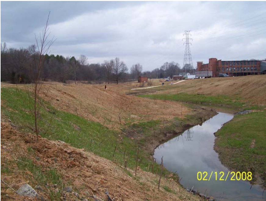
Project looking upstream near Photo Point 23
