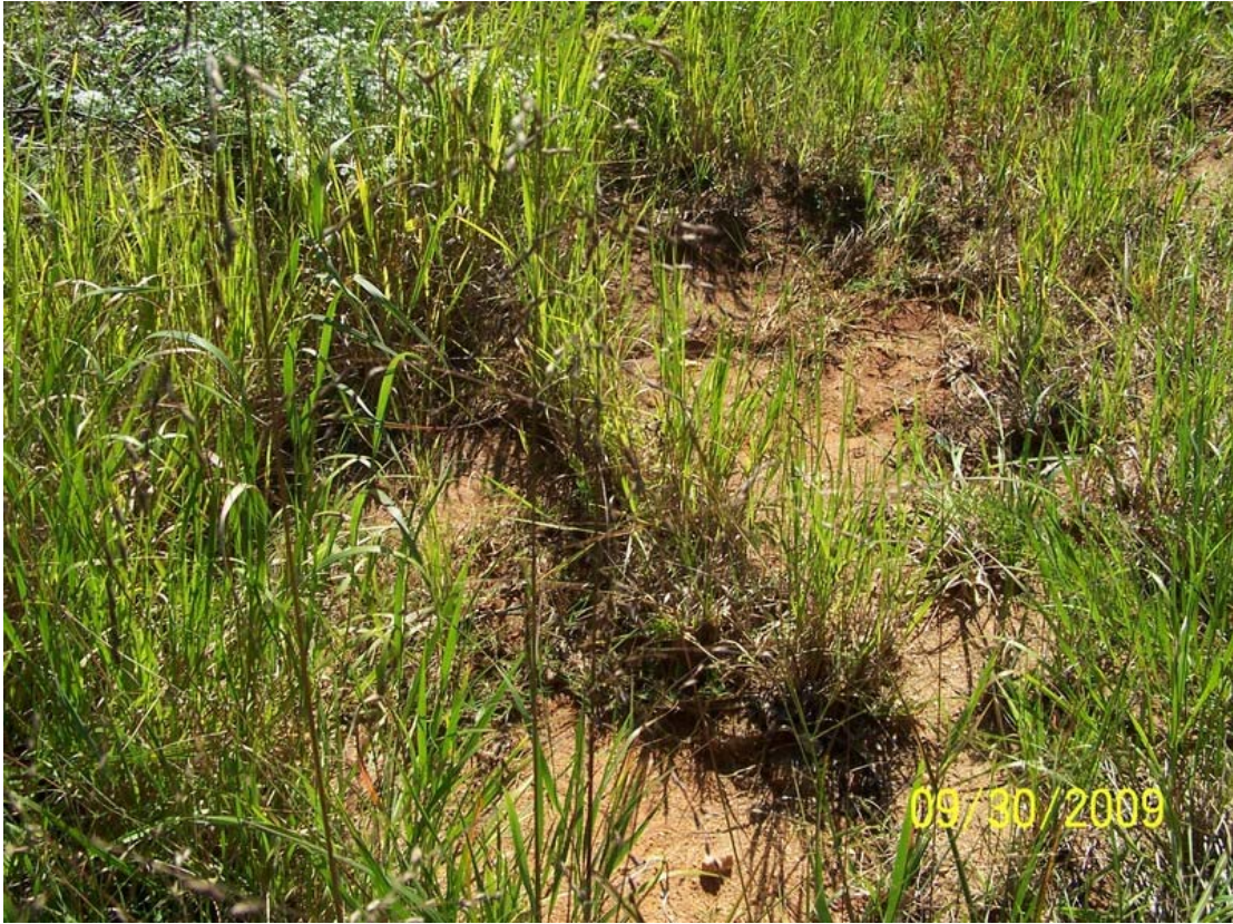
Small scour hole on XS 5, right bank
