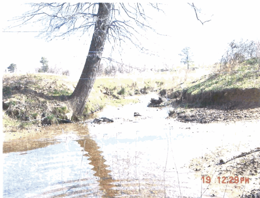
Photo 1b: View of the first 800 feet of the project reach near first ford crossing, looking downstream.
