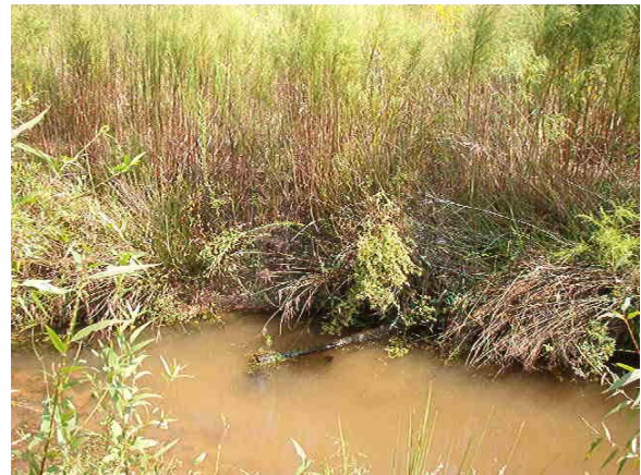
Photo 12, bank scour at station 19+10
