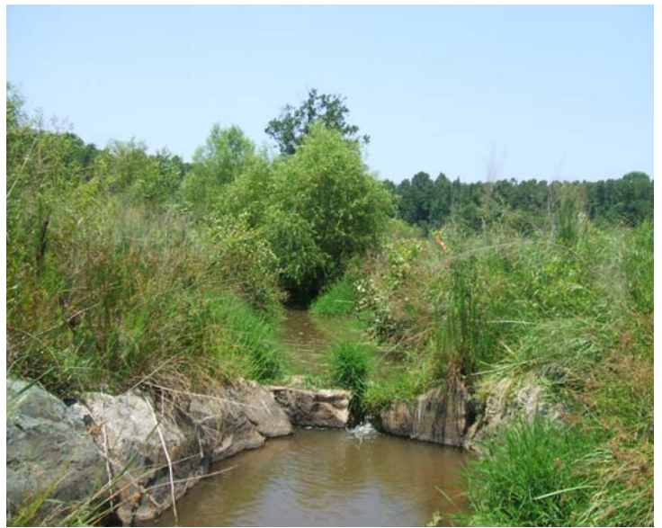
Station 11+30 looking upstream
