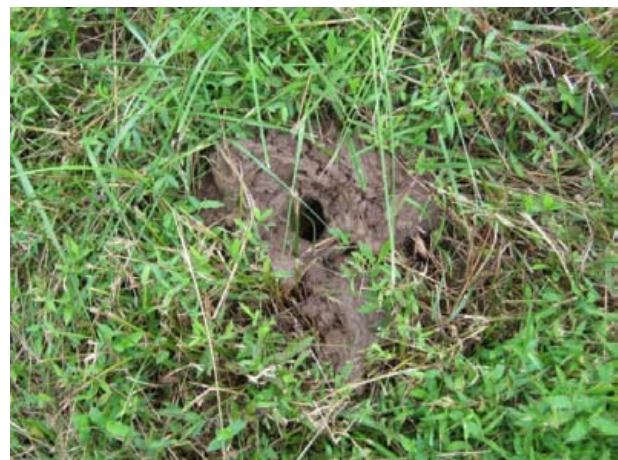
Among many, a crawfish hole located on Site.
