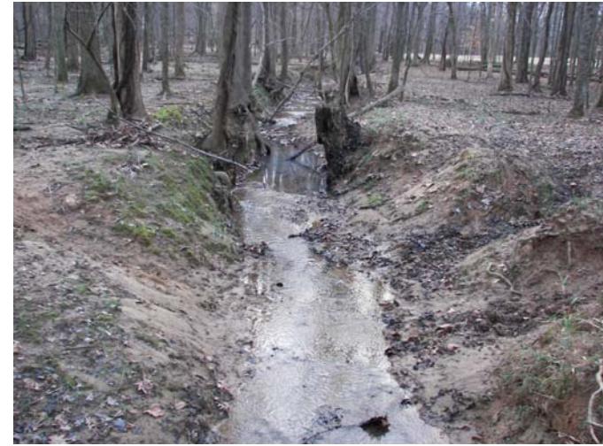
23. Unnamed Tributary Bank Slump 1.2.2007
