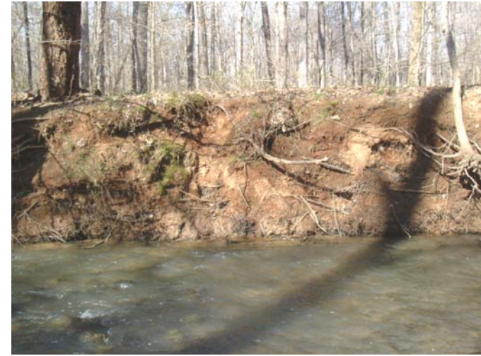
2. Main Channel Vertical, Bare Bank 1.11.2007
