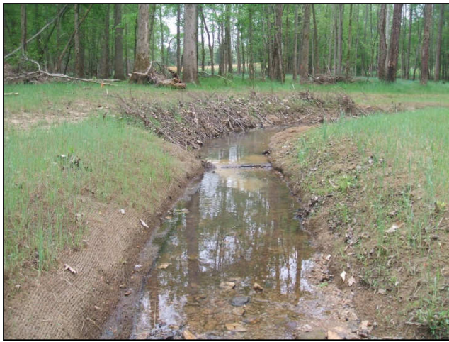
Cross-Section 4-View Upstream Unnamed Tributary (4/2010)
