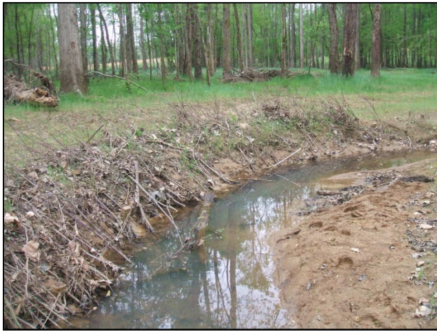
Cross-Section 3-View Upstream Unnamed Tributary (4/2010)
