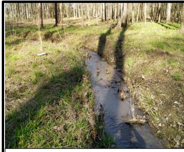
Restored Tributary station 03+00, Photo Point #27, (downstream). 10Apr2014.
