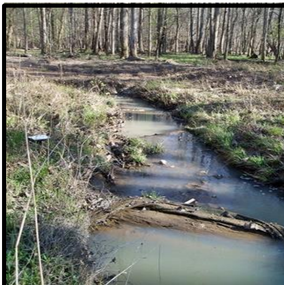
Restored Tributary station 05+40, Photo Point #30, (downstream). 10Apr2014.
