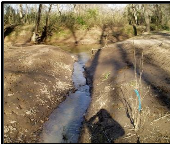
Restored Tributary station 05+80, Photo Point #31, facing E (downstream). Sparse bank vegetation. 10Apr2014.
