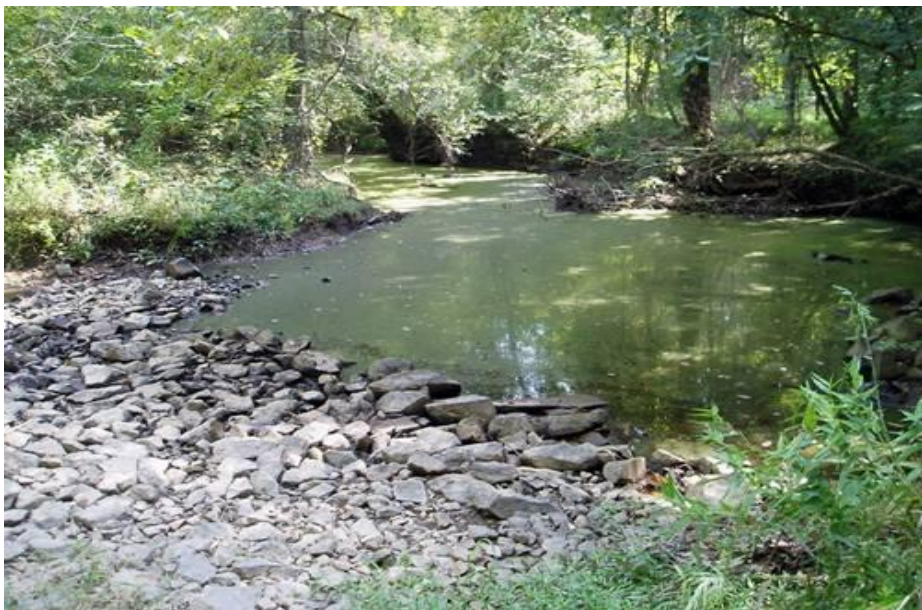
DBC station 94+30 facing upst from rock crossing
