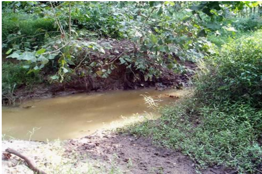
DBC / Tributary confluence: erosion & bed scour, Sep 2015
