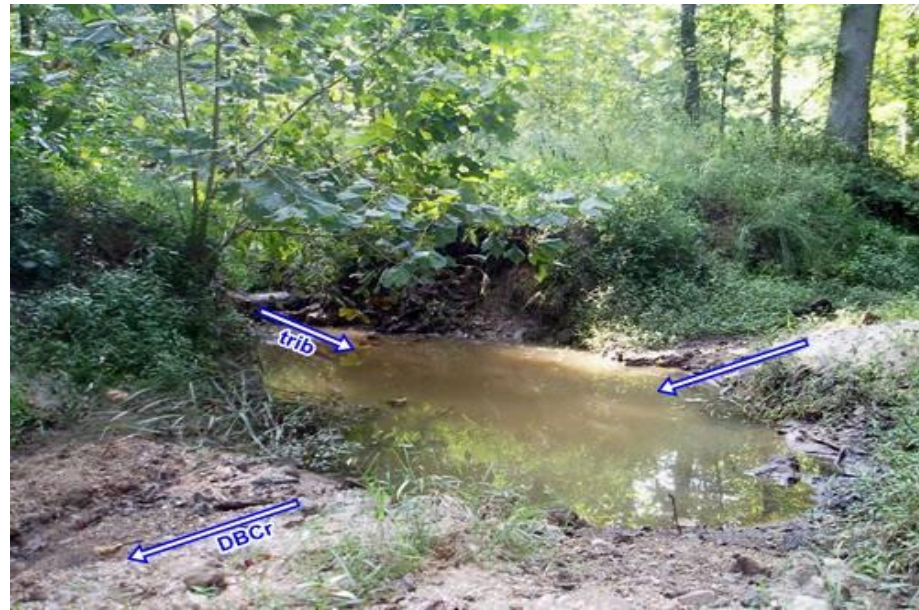
Bed scour in DBC at Trib confluence, face upst, Sep 2015
