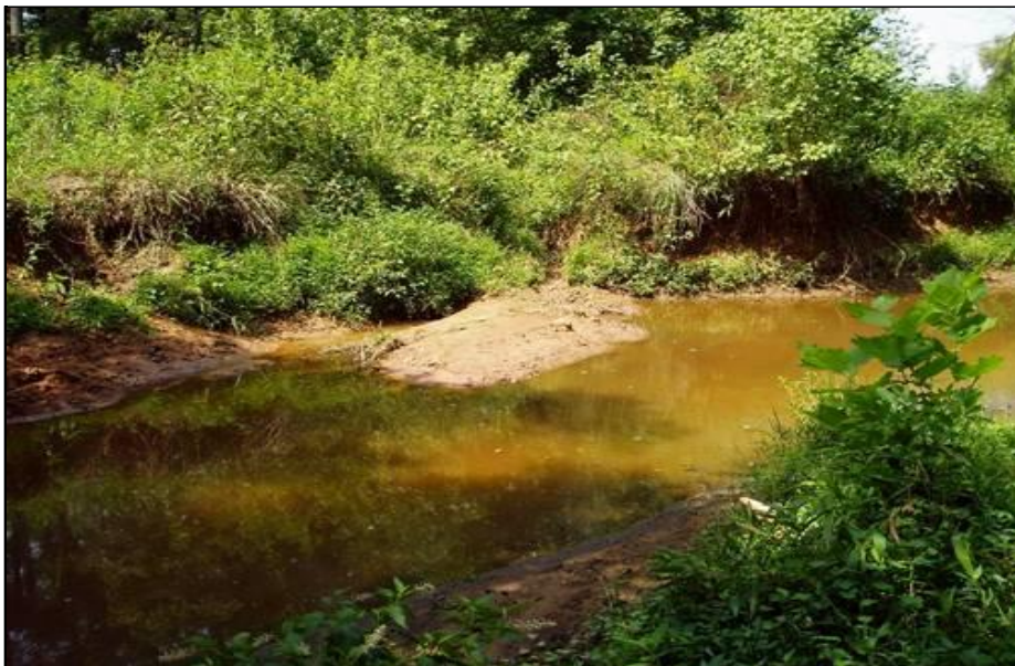
DBC RBK sta 16+80 erosion, face upst, Sep 2015
