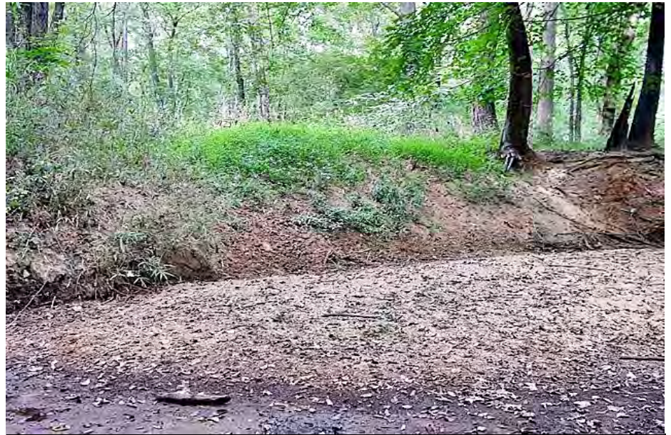
DBC construction crossing, Station 32+50, Sept 2016
