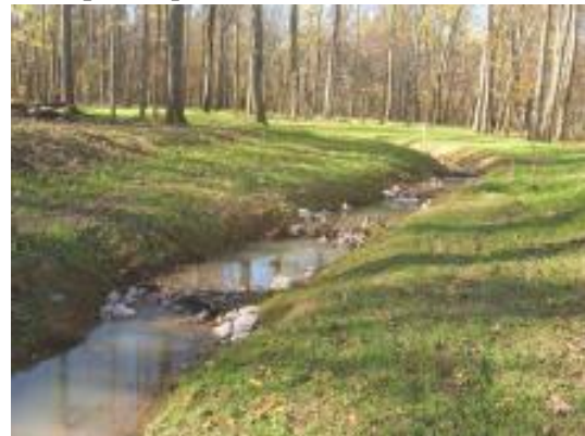
Unnamed Tributary immediately after restoration
