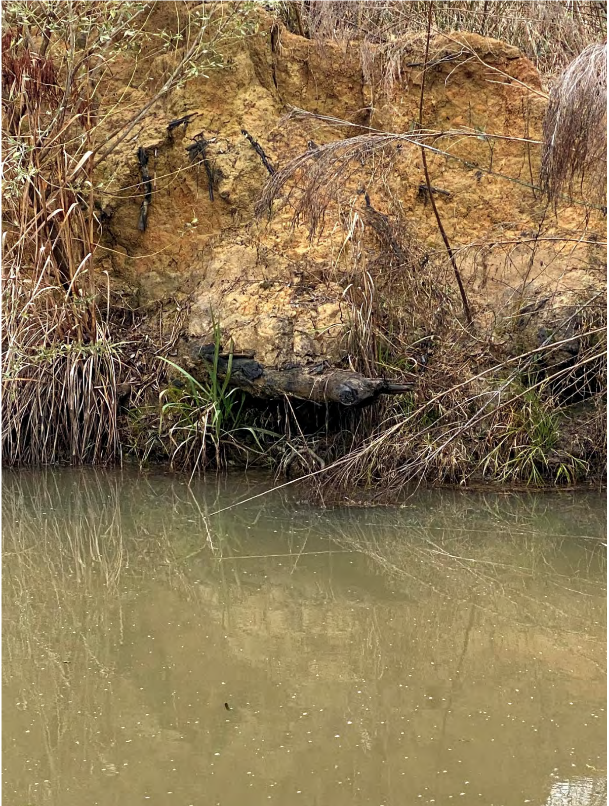
Photo 1.) UT-2 Failed Crossing – Historic floodplain elevation with historic tree roots visible at break between historic floodplain and fill material
