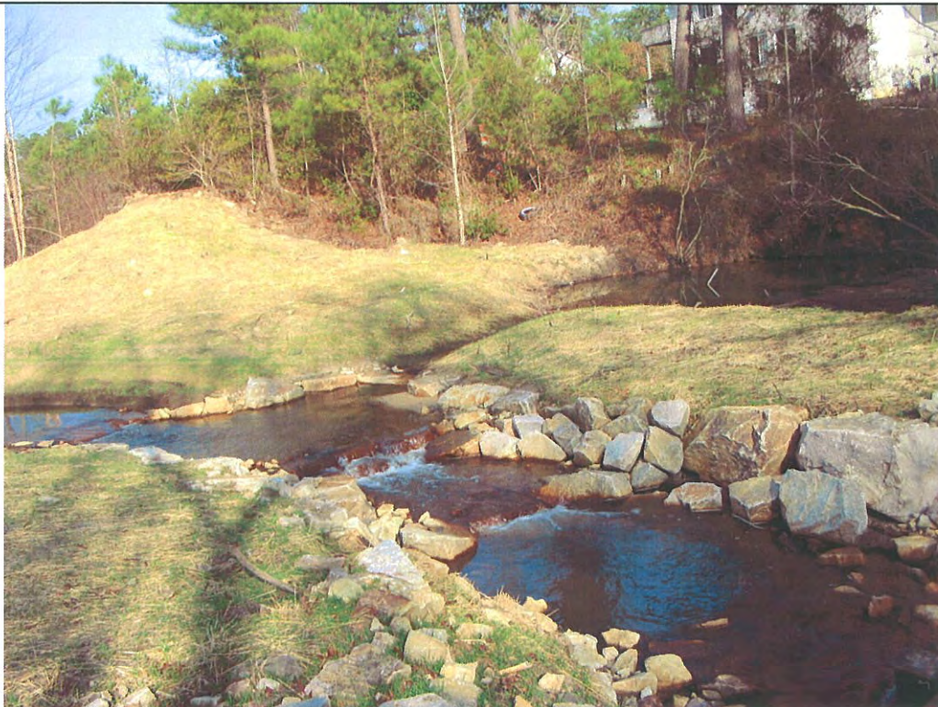
Photograph 4. Phase I Completed: Restored section of stream. Photo taken 1/12/2006.
