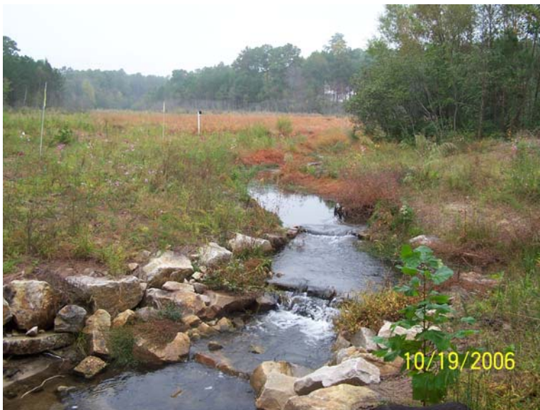
Photo Point 3 – Structures 1 & 2
