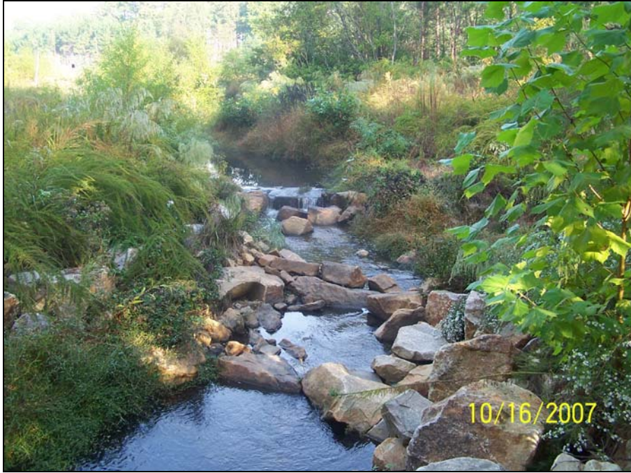
Photo Point 3 – Structures 1 & 2
