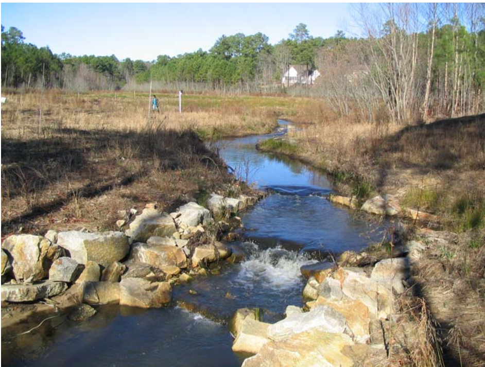
Main Structure after bank full event , January 2007
