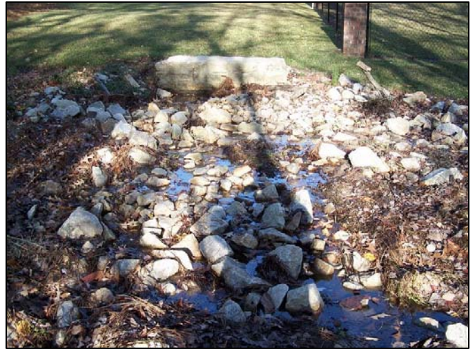
Outfall N of monitoring well CEC10
