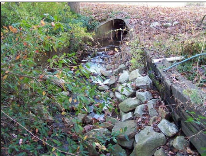
Outfall W of monitoring well TARLTON4
