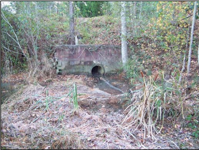
Outfall near Photo Point 1
