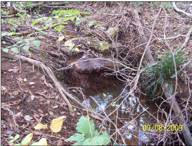
Outfall N of Well CEC10
