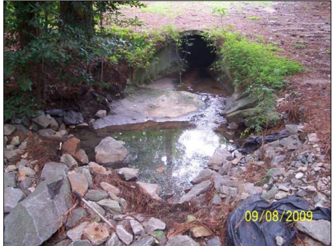
Outfall NW of Well CE2
