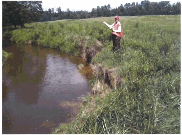
Outer Bend #24 - Looking Upstream at a short reach of erosion. (Severe Erosion)
