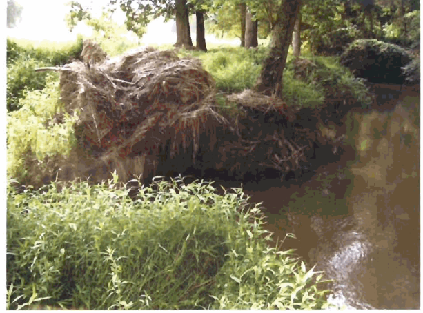
Outer Bend #11 - Looking Downstream at fallen tree causing a hole in the bank. (Severe Erosion)
