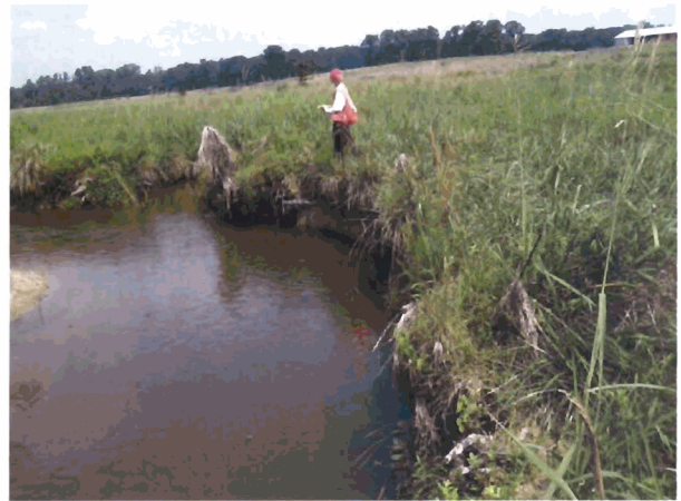
Outer Bend #19 - Looking Upstream (Severe Erosion)
