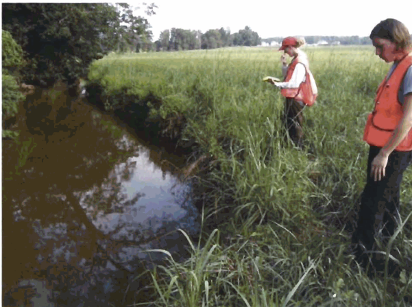
Outer Bend #9 - Looking Upstream at outer bend in a straight, immediately upstream from a tight radius. (Moderate Erosion)
