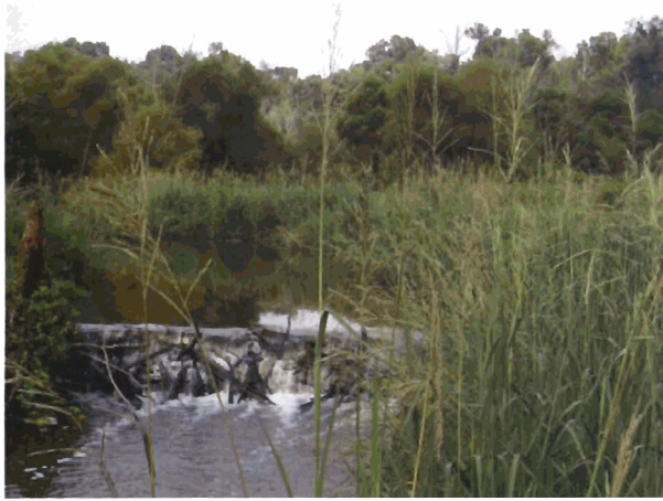
Outer Bend #1 - Looking Upstream at beaver dam. (Low Erosion)
