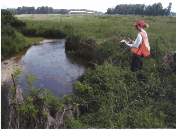
Outer Bend #17 - Looking Upstream (Severe Erosion)
