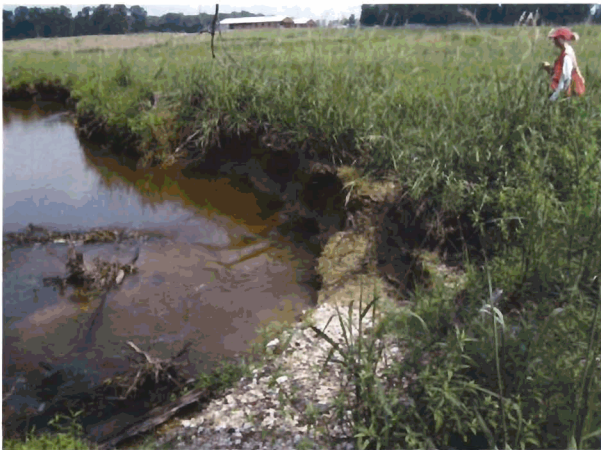
Outer Bend #18 - Looking Upstream (Extreme Erosion)
