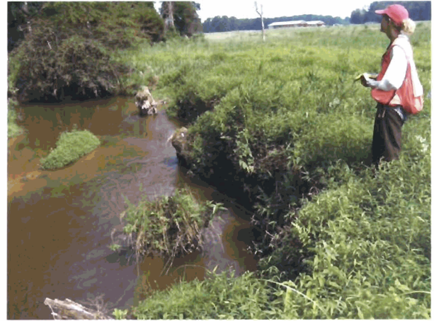
Outer Bend #15 - Looking Upstream at a long bend with two stumps extending into the stream. (Moderate Erosion)
