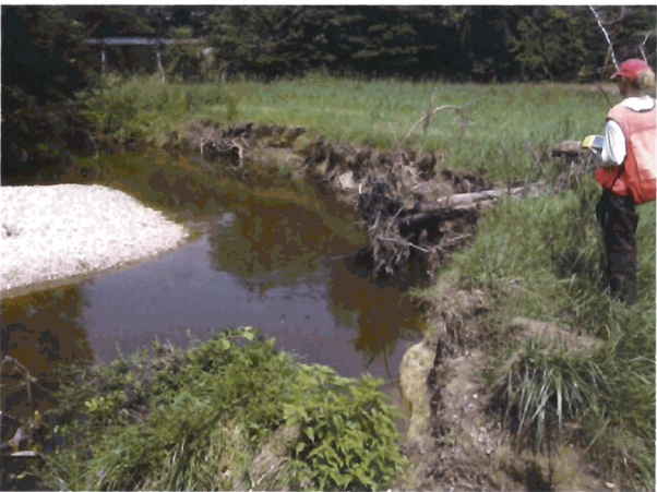
Outer Bend #30 - Looking Upstream at lateral migration of out bend with extension of point bar into the stream bed. (Extreme Erosion)
