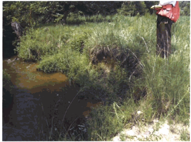
Outer Bend #29 - Looking Upstream at shoot cutoff. Not a good bank erosion treatment comparison area. (Severe Erosion)
