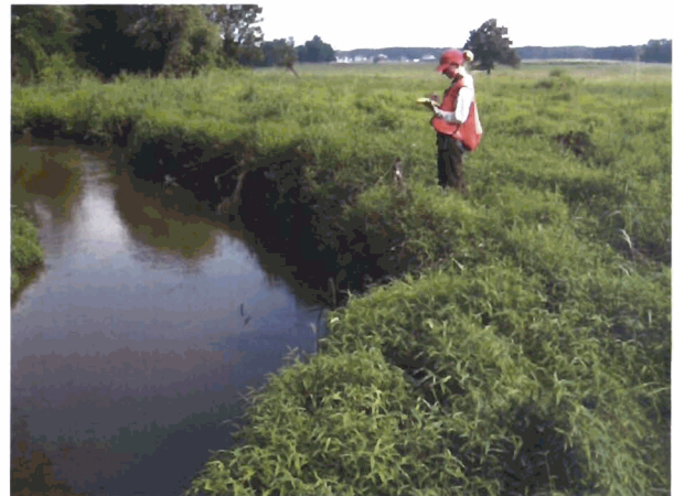
Outer Bend #6 - Looking Upstream in a double outer bend. (Moderate Erosion)
