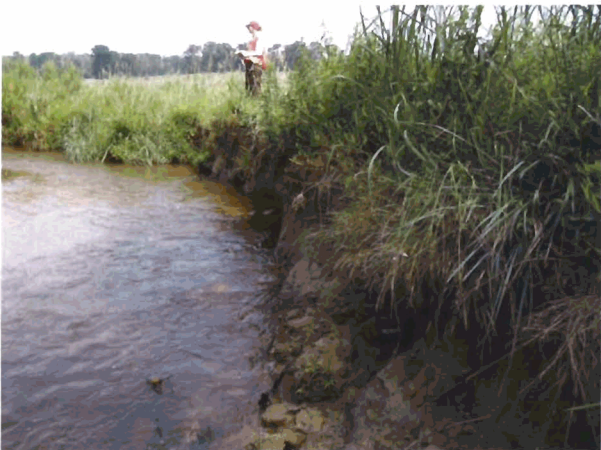
Outer Bend #20 - Looking Upstream at a long bend with a tight radius in the middle of the bend. (Extreme Erosion)
