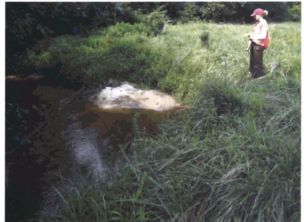
Outer Bend #13 - Looking Upstream A fallen tree may be causing erosion on Site stream banks. (Severe Erosion)
