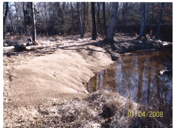
Outer Bend 12 (Live stake with erosion control matting)
