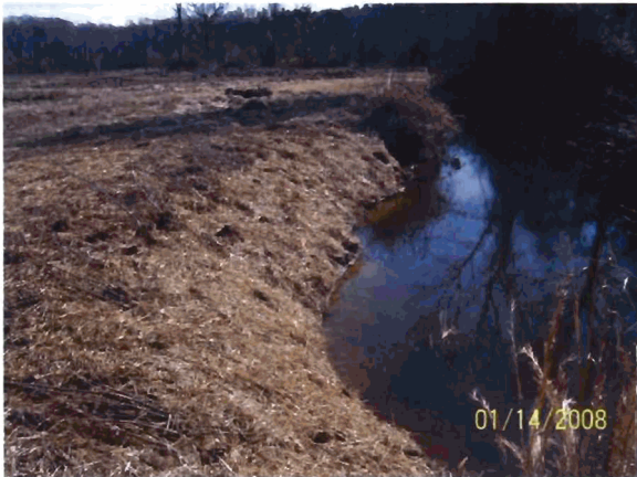
Outer Bend 8 (Live stake with erosion control matting)
