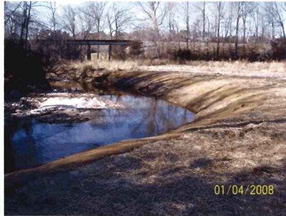
Outer Bend 30 (Live stake with erosion control matting)
