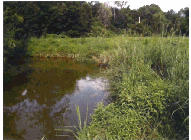
Outer Bend #4 - Looking Upstream approximately 500 ft upstream from beaver dam, still in impounded reach. (Moderate Erosion)
