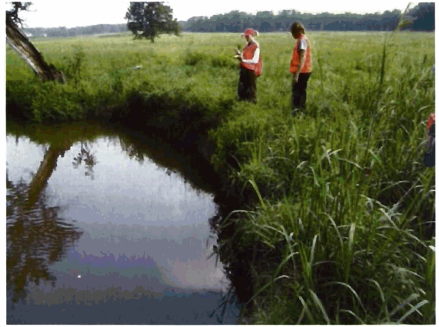
Outer Bend #8 - Looking Upstream (Severe Erosion)
