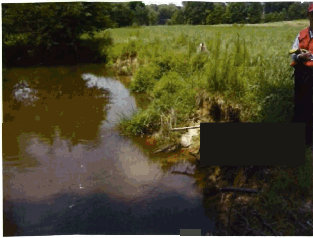
Outer Bend #27 - Looking Upstream at erosion on low slope reach. (Severe Erosion)
