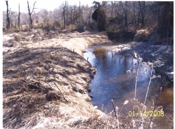
Outer Bends 6 (Live stake with erosion control matting) and 7 (Brush Mattress)
