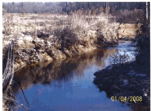
Outer Bend 19 (No Treatment)
