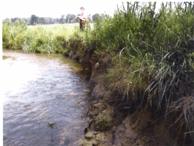
Outer Bend #20 - Looking Upstream at a long bend with a tight radius in the middle of the bend. (Extreme Erosion)
