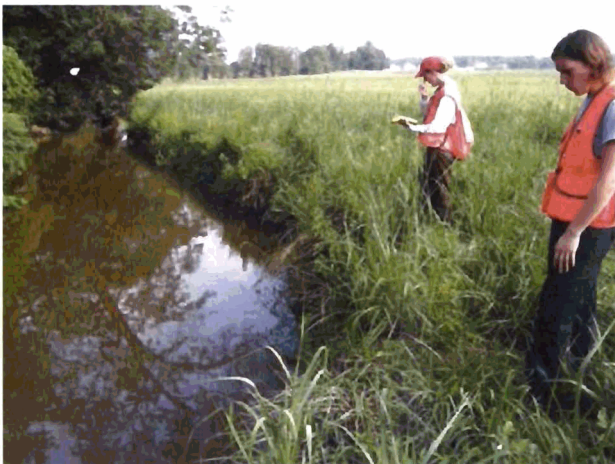
Outer Bend #9 - Looking Upstream at outer bend in a straight, immediately upstream from a tight radius. (Moderate Erosion)
