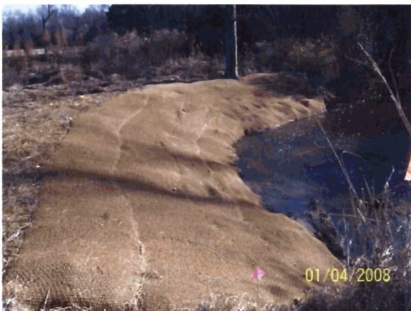
Outer Bend 18 (Live stake with erosion control matting)
