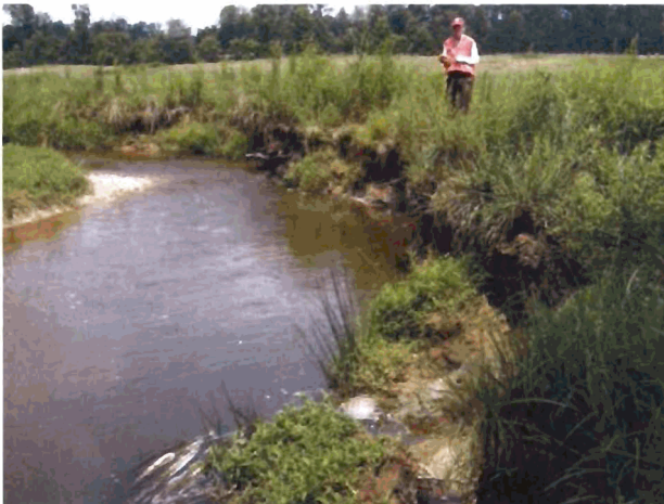
Outer Bend #25 - Looking Upstream at transverse bar and tight radius at upper reach of the bend. (Extreme Erosion)
