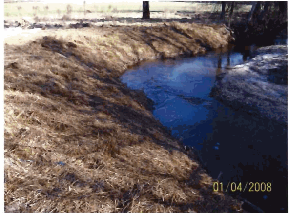
Outer Bend 15 (Live stake with erosion control matting)
