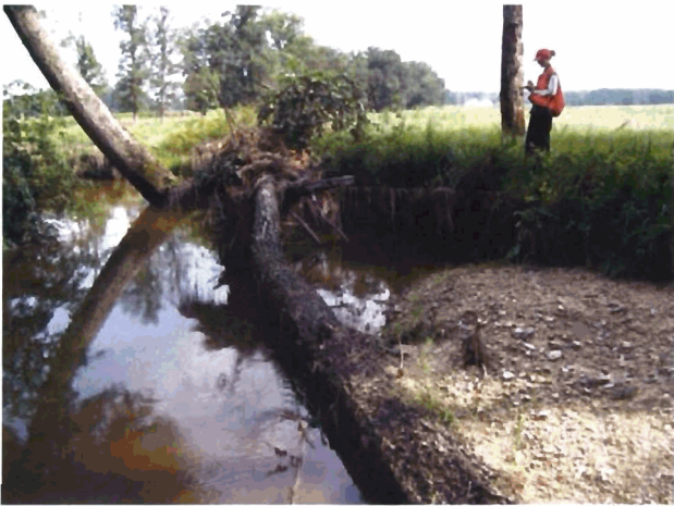
Outer Bend #12 - Looking Upstream (Severe Erosion)
