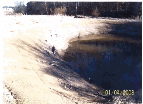
Outer Bend 28 (Live stake with erosion control matting)
