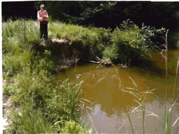
Outer Bend #28 - Looking Downstream at potential shoot cutoff development. (Severe Erosion)
