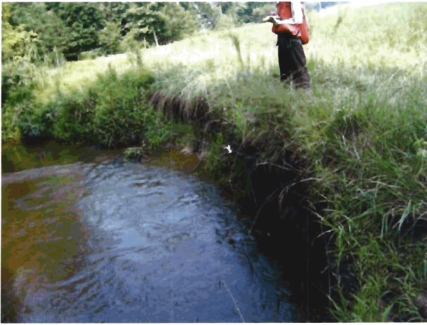
Outer Bend #14 - Looking Upstream at tight radius caused by point bar and transverse bar. (Severe Erosion)
