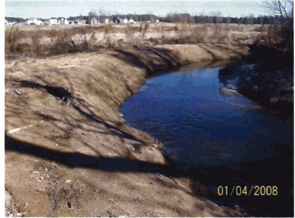
Outer Bend 22 (Live stake with erosion control matting)
