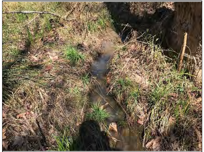
PP-38: Reach 6, view upstream at Station 11+50
