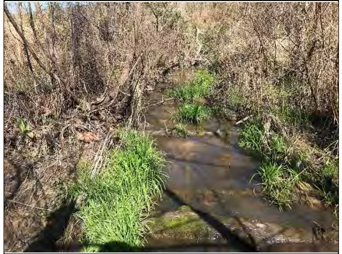
PP-20: Reach 2, view upstream at Station 23+00
