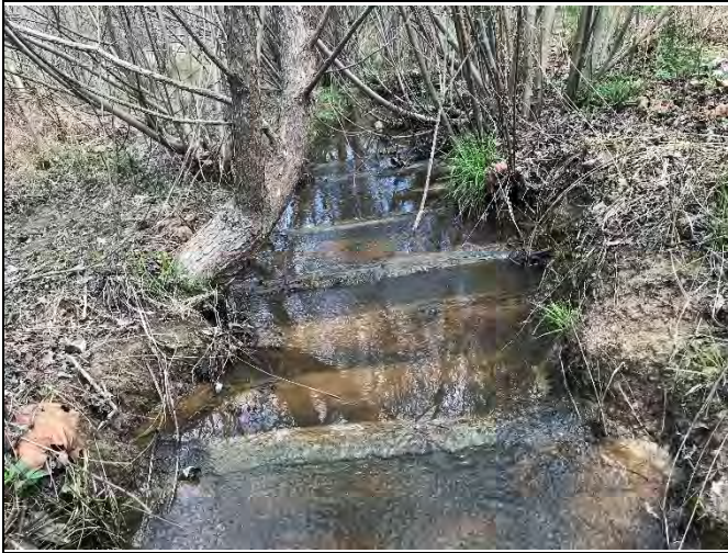
PP-55: Reach 5, view downstream at Station 37+30
