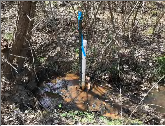
PP-51: Reach 5, Flow Gauge #2 at Station 33+90
