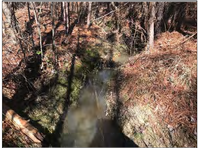
PP-40: Reach 6, view upstream at Station 18+90
