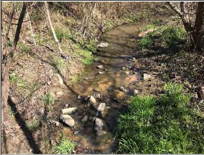
PP-19: Reach 2, view upstream at Station 22+00
