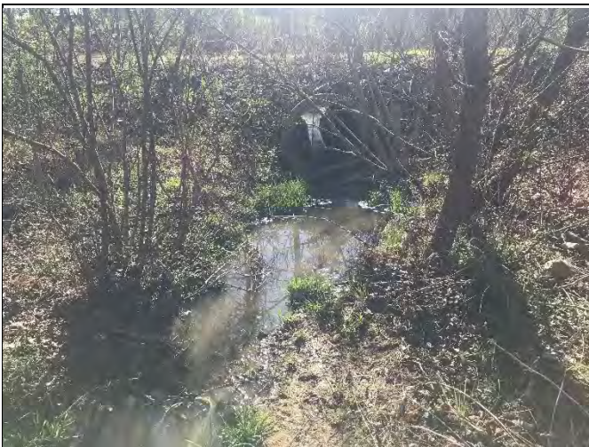
PP-5: Reach 3, view downstream towards pipe crossing, Station 18+50
