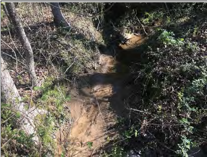
PP-11: Reach 4, view upstream at Station 10+10
