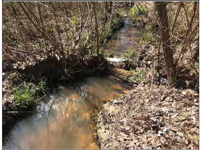
PP-46: Reach 5, view downstream at Station 30+75
