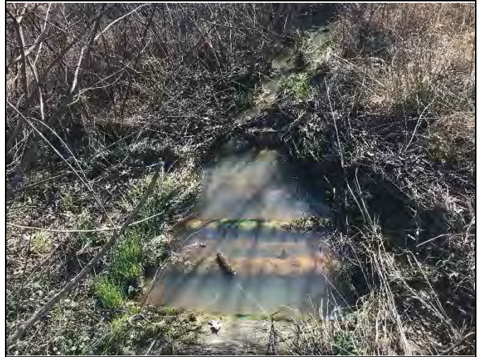
PP-4: Reach 3, view downstream, Station 16+25
