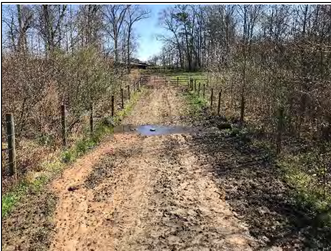
PP-23: Reach 2, view of crossing at Station 27+75
