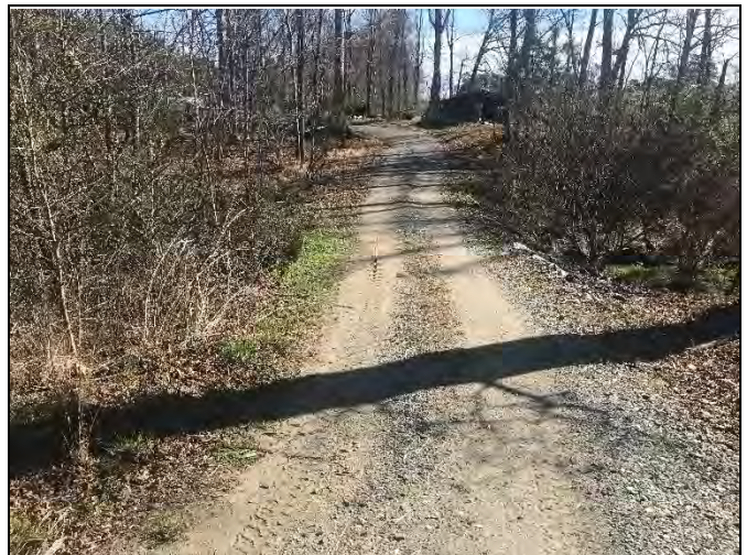
PP-6: Reach 3, stream crossing, Station 18+80
