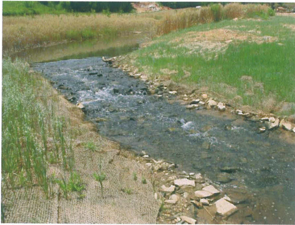
Photograph No. 7- Riffle at Station 25+84 on Mainstem, Looking Upstream
