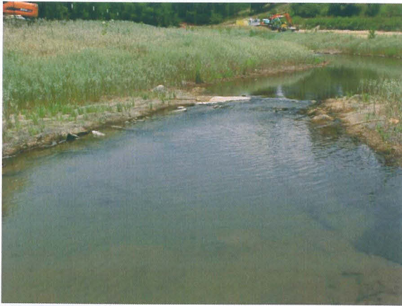
Photograph No. 9- J-Hook at Station 15+80 on Mainstem, Looking Upstream
