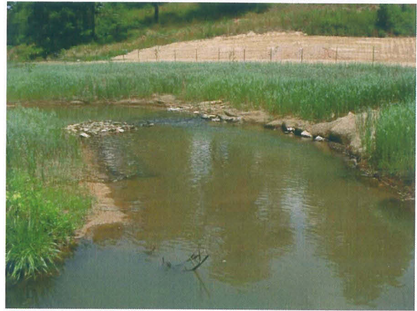
Photograph No. 10- J-Hook at Station 9+95 on Mainstem, Looking Upstream
