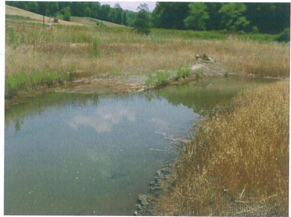
Photograph No. 8- Log Vane at Station 23+40 on Mainstem, Looking Downstream
