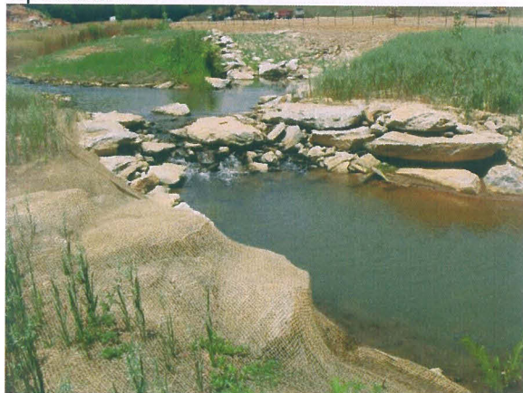
Photograph No. 6- Cross Vane at Station 26+45 on Mainstem, Looking Upstream
