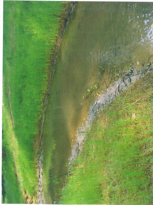
Cross-section photo – looking downstream
