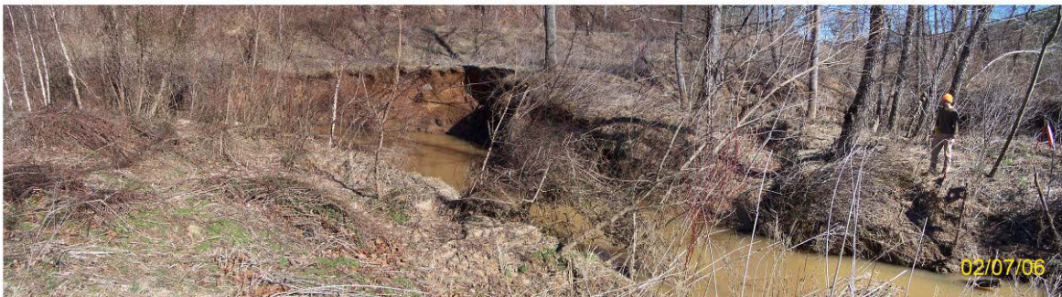
Thompsons Fork Mainstem – Pre-Restoration Photograph taken near downstream limits of project. 15-ft Vertical to Undercut Stream Bank
