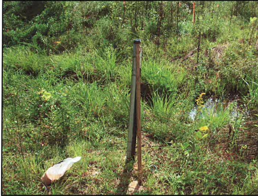
BF 1 Crest Gage at XS-6 on UT. (EMH&T, Inc. 9/21/09)
