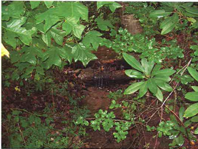
Cross-section photo – looking upstream
