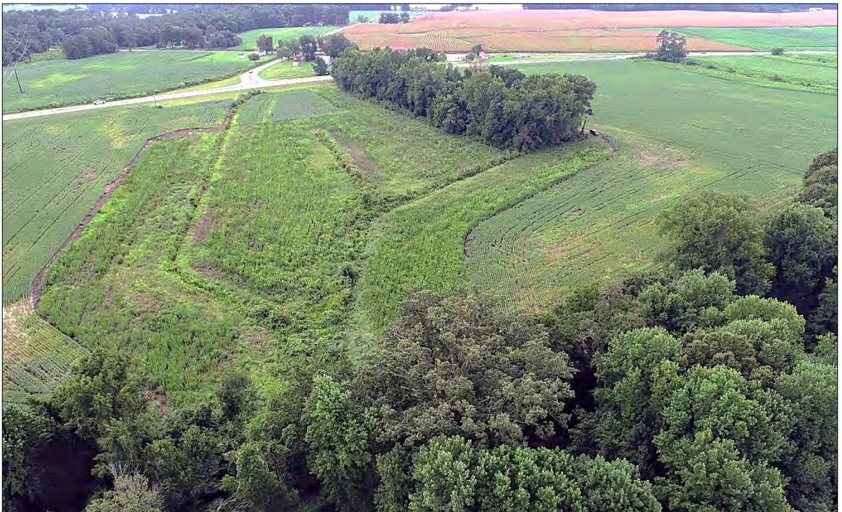
Photo 2 – Features 1A, 1B, 2, and 3 (Looking south w/ Hwy. 55 in the background) Photo Date, August 16, 2022
