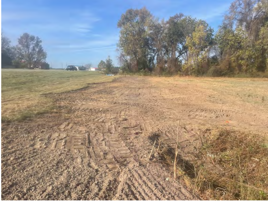
Photo 1: Upper portion of Feature 1C (ditch) filled in, facing west. November 9, 2022
