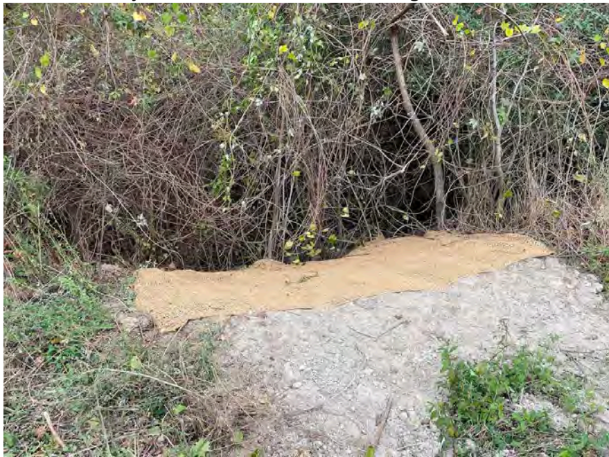
Photo 6: Ditch adjacent to Feature 2 filled in, facing west. November 9, 2022
