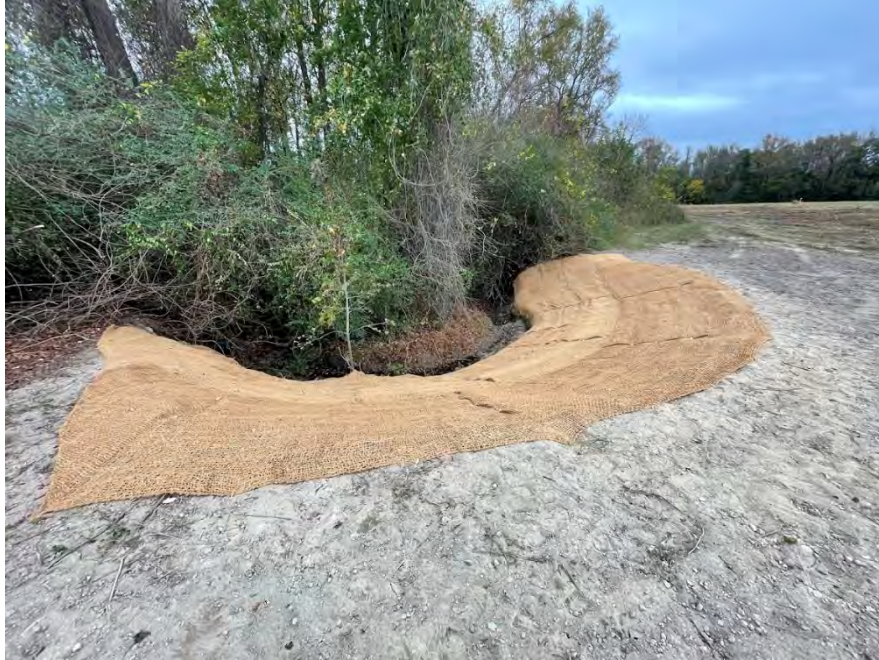
Photo 5: Bank Stabilization on Feature 4, facing north. November 9, 2022
