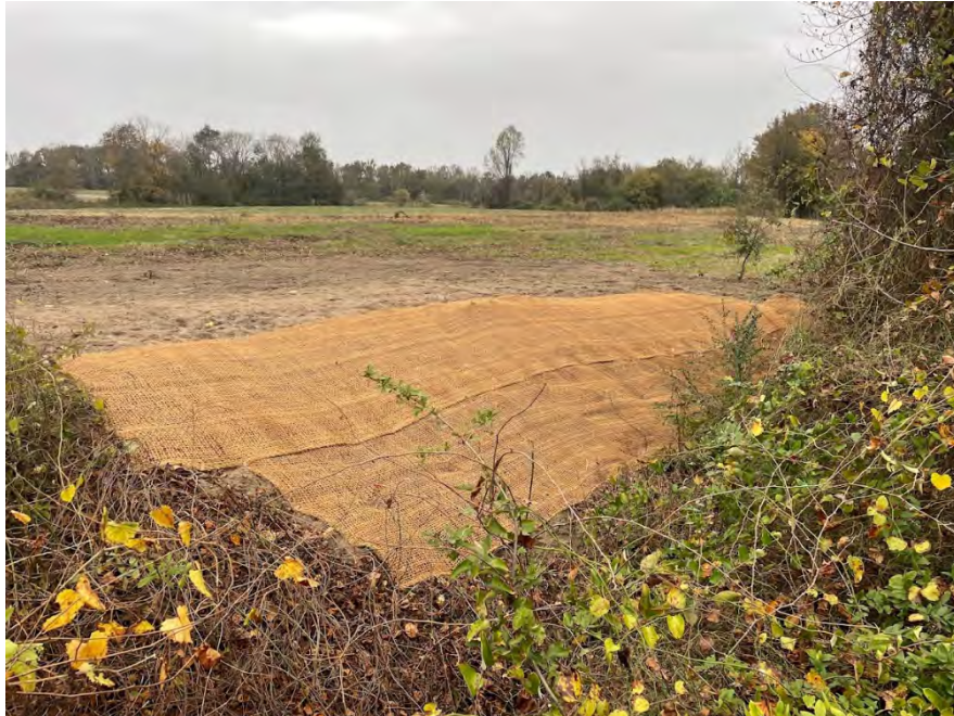
Photo 10: Bank Stabilization on Feature 5, facing northwest. November 9, 2022
