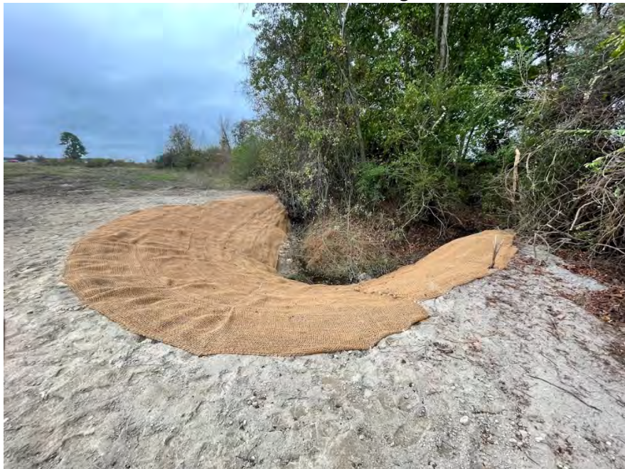
Photo 4: Bank Stabilization on Feature 4, facing south. November 9, 2022
