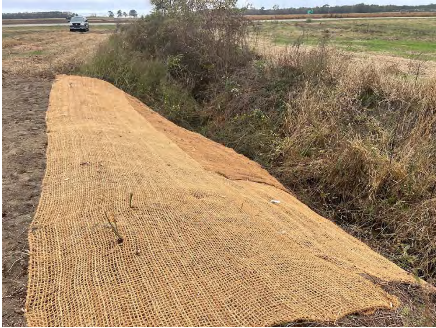
Photo 9: Bank Stabilization on Feature 5, facing south. November 9, 2022
