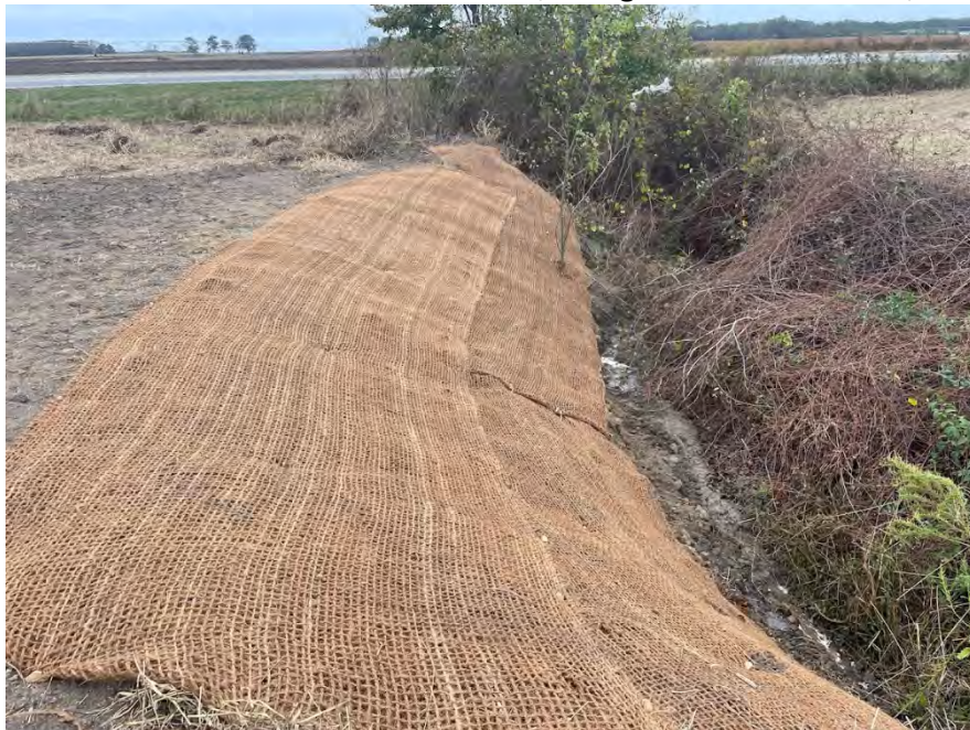
Photo 8: Bank Stabilization on Feature 5, facing south. November 9, 2022
