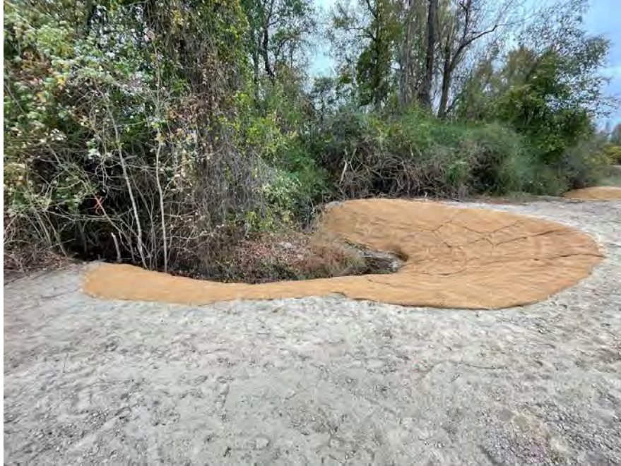
Photo 3: Bank Stabilization on Feature 4, facing north. November 9, 2022
