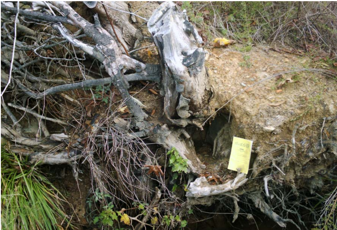
SP4. Lateral bankcut in rootwad
