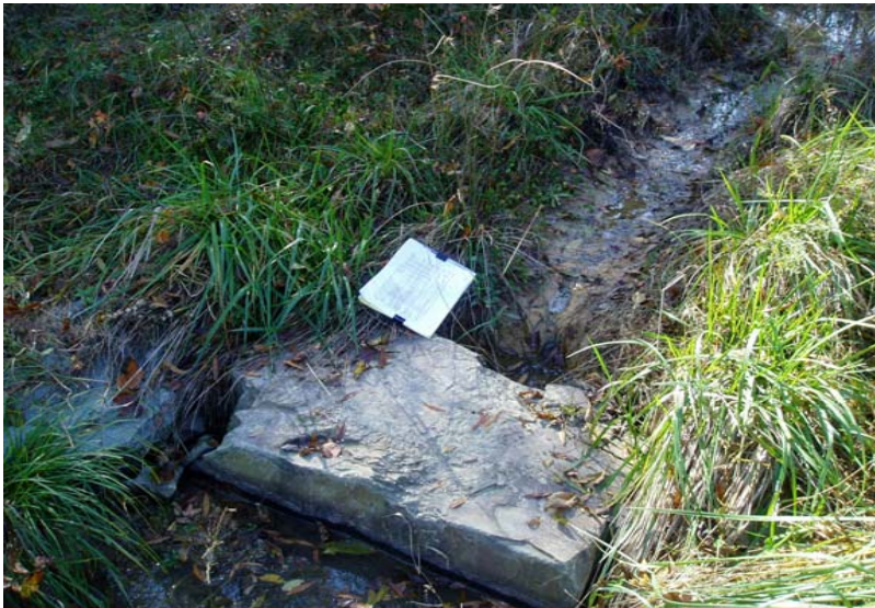
SP3 - Backcut and piping (11/11/2008)
