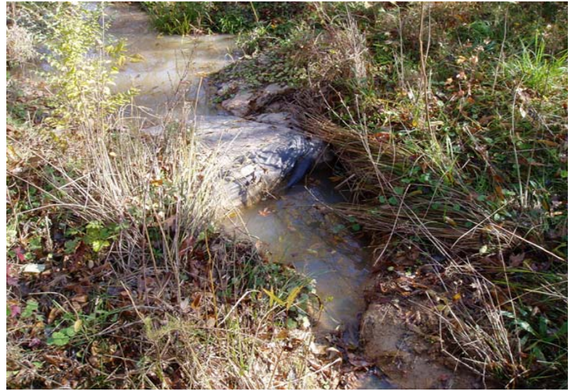
SP2 - Backcut and piping (11/11/2008)
