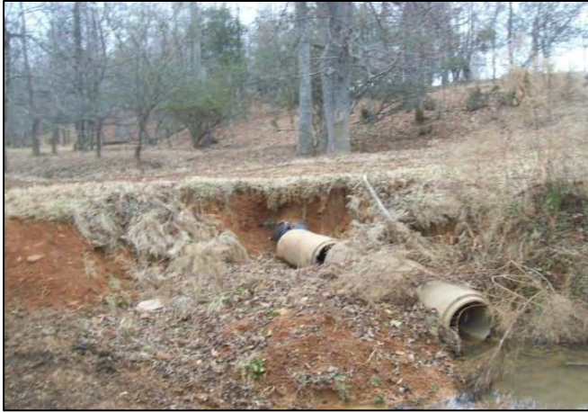
Reach 5 (1-5-11), old crossing at 41+75
