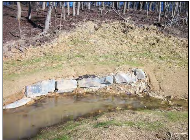
PID 20: Station 23+60 – Left Bank (12/15/15)
