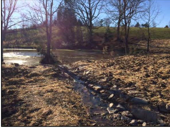
PID 41: Station 47+00 – Right Floodplain Rock Lined Channel from Wetland (1/13/16)
