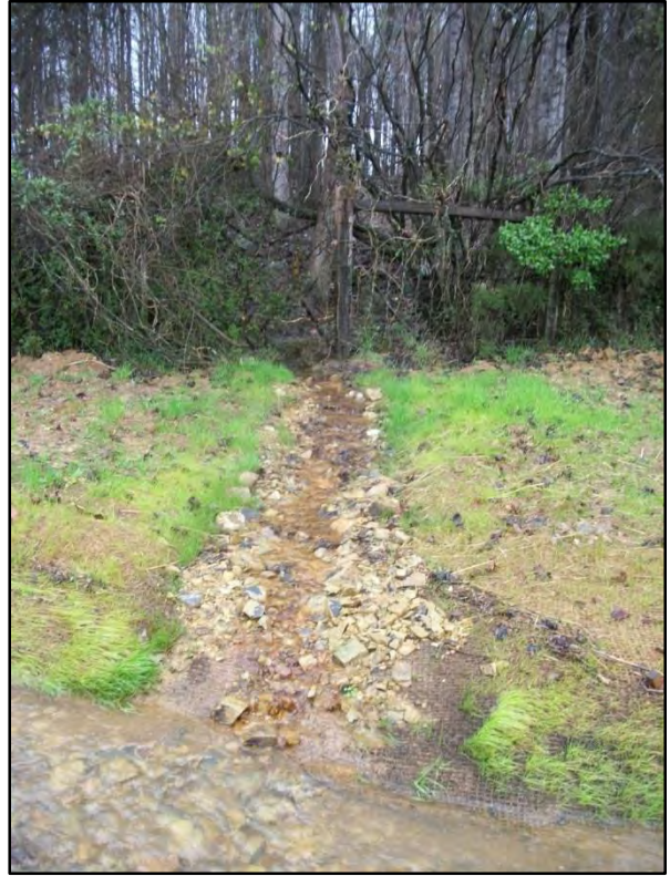
PID 3: Station 10+70 – Left Floodplain Rock Lined Channel (12/31/15)
