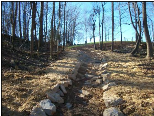
PID 25: Station 28+35 – Right Floodplain Rock Lined Channel (1/13/16)
