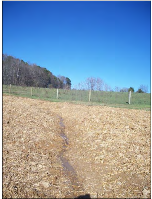
PID 8: Station 14+65 – Left Floodplain Matted Drainage Swale (1/14/16)
