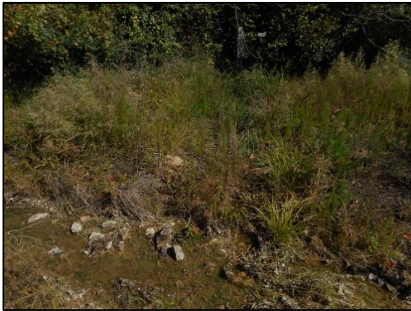
PID 3: Station 10+70 – Left Floodplain Rock Lined Channel (10/12/16)
