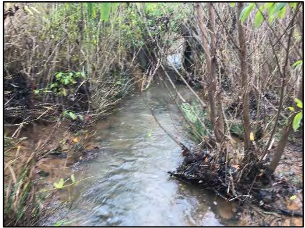
PID 38: Station 45+30 Downstream (11/14/18)
