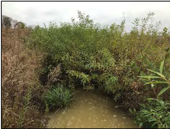
PID 9: Station 14+65 – Downstream (11/14/18)
