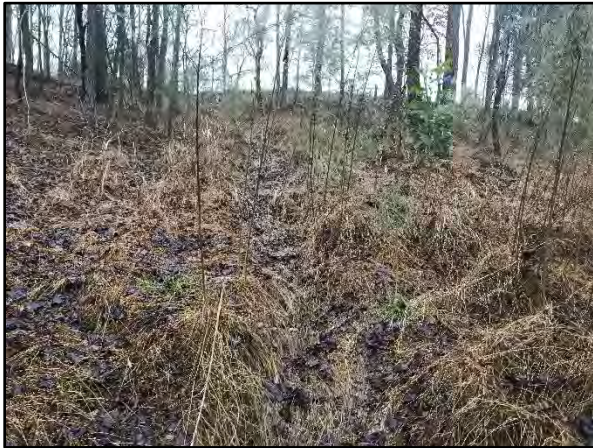
PID 25: Station 28+35 – Right Floodplain Rock Lined Channel (11/14/18)
