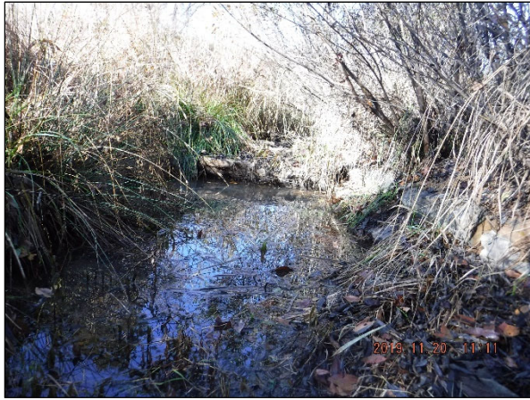
PID 19: Station 23+60 – Upstream (11/20/19)
