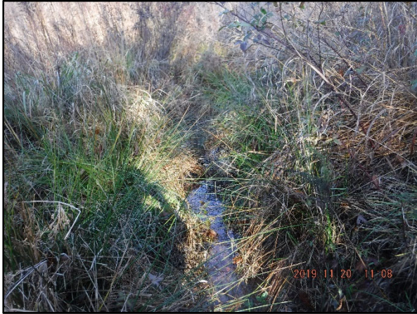
PID 17: Station 21+75 – Upstream (11/20/19)
