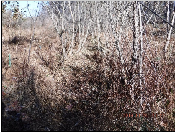
PID 25: Station 28+35 – Right Floodplain Rock Lined Channel (11/20/19)
