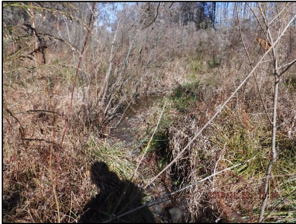
PID 31: Station 35+50 – Upstream (11/20/19)
