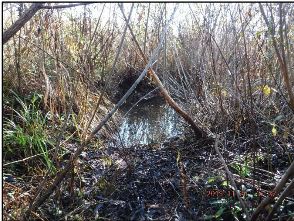
PID 3: Station 10+70 – Left Floodplain Rock Lined Channel (11/20/19)
