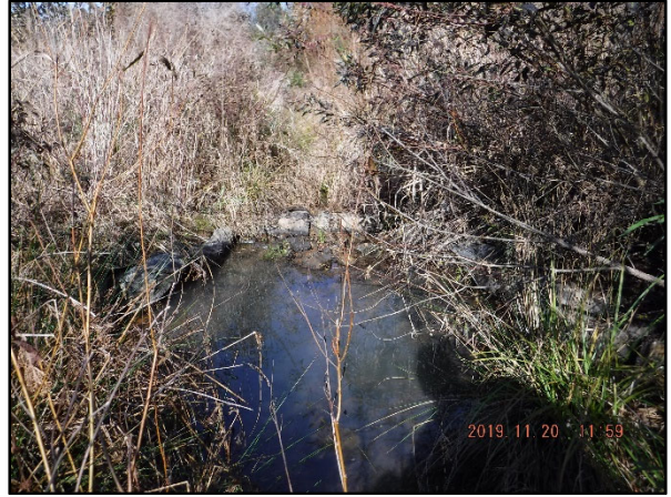
PID 42: Station 47+75 – Upstream (11/20/19)
