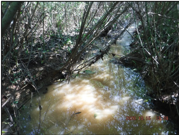
PID 3: Station 10+70 – Left Floodplain Rock Lined Channel (10/15/20)
