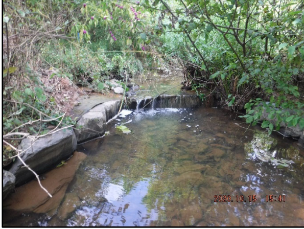
PID 41: Station 47+00 – Right Floodplain Rock Lined Channel from Wetland (10/15/20)
