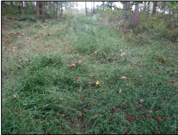
PID 25: Station 28+35 – Right Floodplain Rock Lined Channel (10/15/20)
