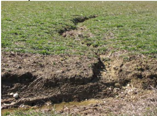
Photo 11: Rill erosion on Tributary 3: February 2010
