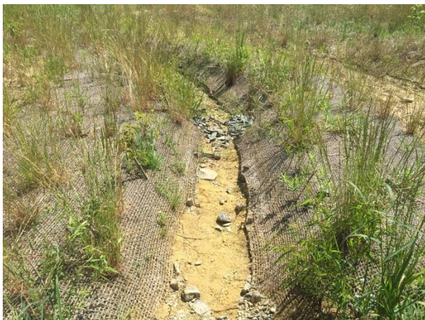
Cross Section 3 (looking upstream) – 6/5/15
