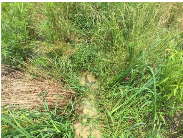
Cross Section 9 (looking upstream) – 6/5/15
