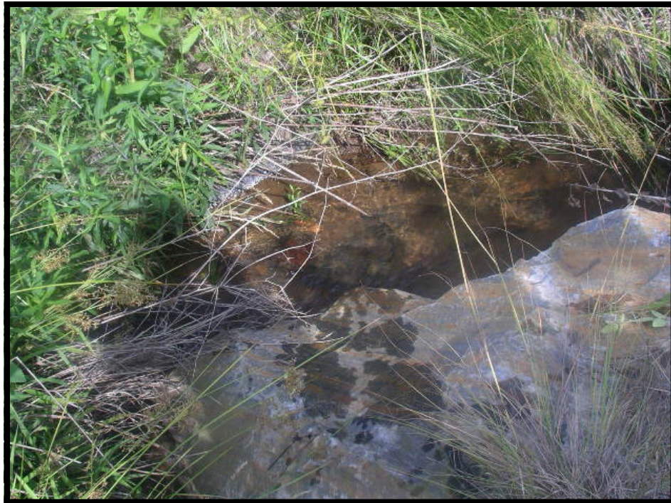
Figure 5—Typical Bank Scour (June 12, 2007)
