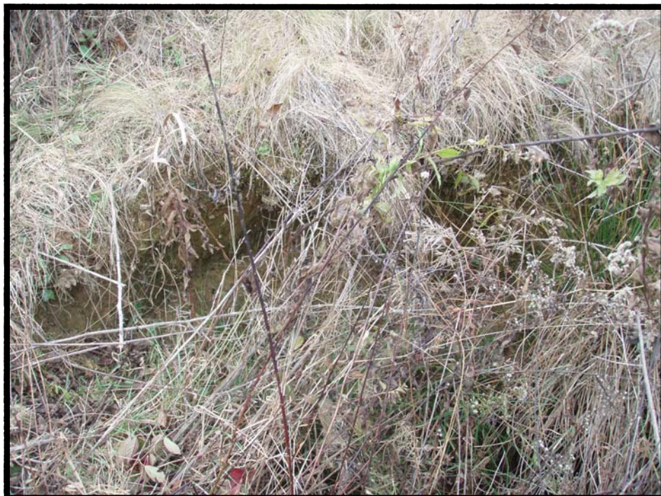
Figure 4—Typical Bank Scour (November 13, 2007)
