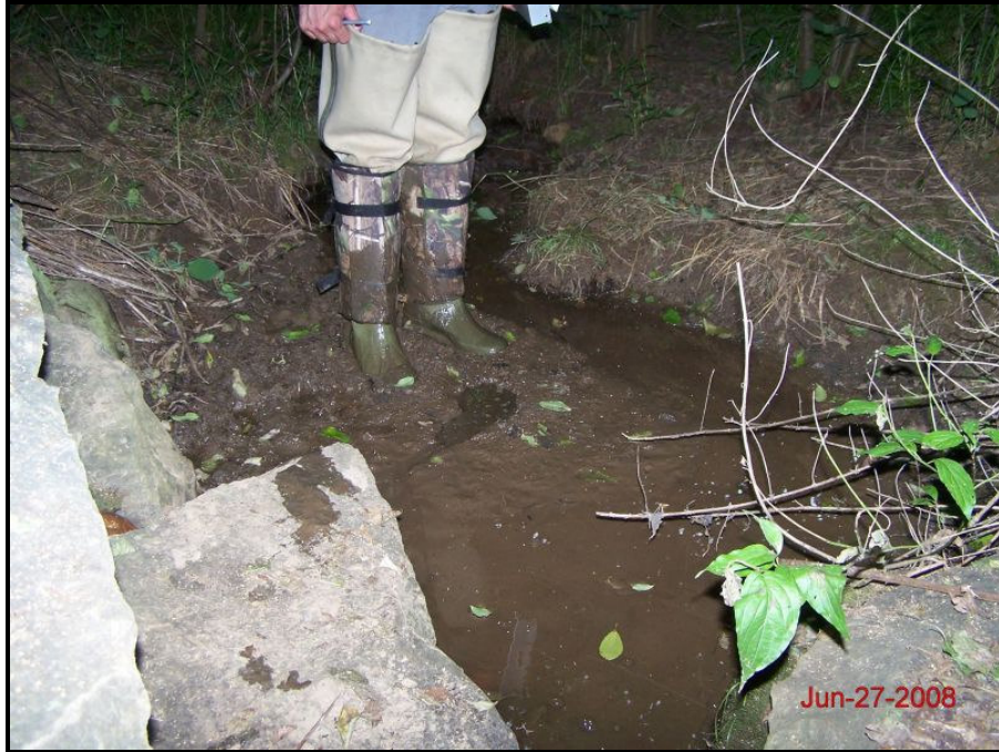
Stream Problem Area (SPA 1) – Pool aggradation Monitoring Year 4 – June 27, 2008
