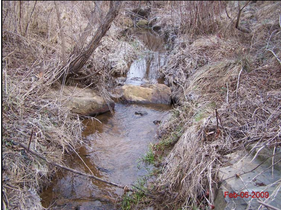
Stream Problem Area (SPA 3) – Stressed Structure Monitoring Year 5 – February 6, 2009
