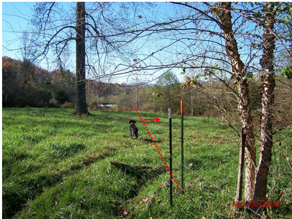
Vegetation Problem Area (VPA 2) – Livestock Encroachment Monitoring Year 5 – November 6, 2009
