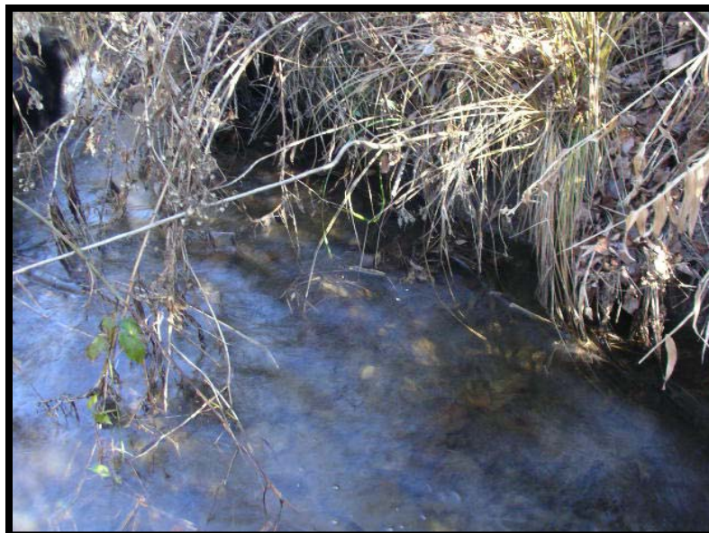
Figure 6—Typical Bank Scour
