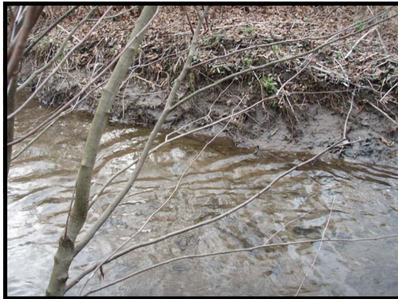
Figure 1—Typical Bank Scour (November 13, 2007)
