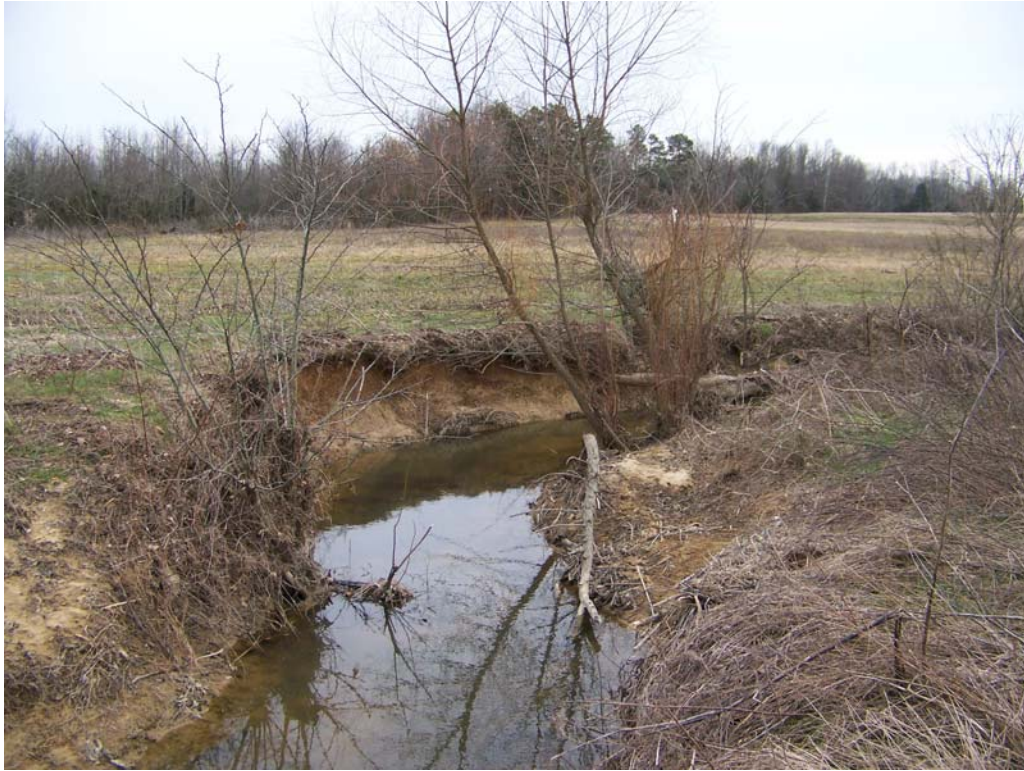
Existing Conditions Reach SF 4
