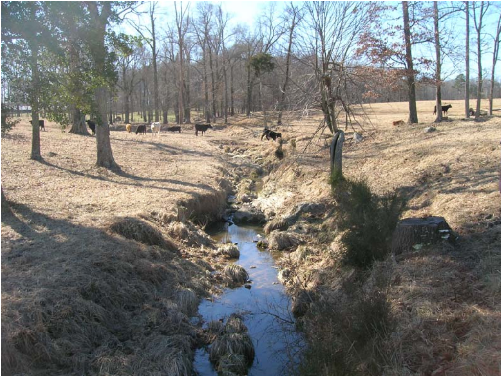
Existing Conditions Reach UT 1
