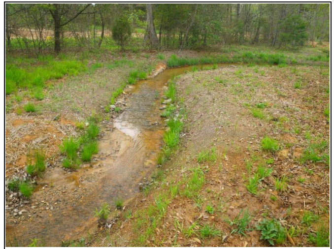
Photo 45. UT3 Photo Point 6 – Station 4+55 (April 17, 2015) downstream from right bank.
