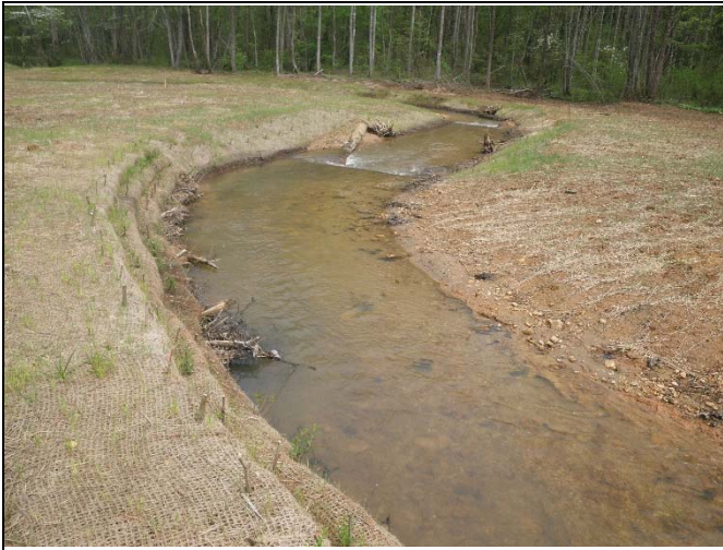
Photo 3. Mainstem Photo Point 2 – Station 26+44 (April 17, 2015) downstream view from left bank.
