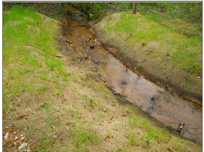
Photo 47. UT3 Photo Point 8 – Station 2+67 (April 17, 2015) upstream to structure.
