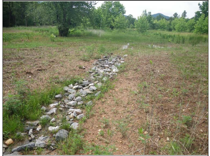
Photo 67. As-built Wetland Photo Point – up valley from left bank at station 22+00.
