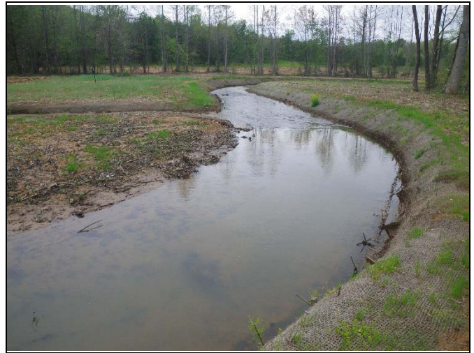
Photo 16. Mainstem Photo Point 8 – Station 5+06 (April 17, 2015) downstream from right bank.
