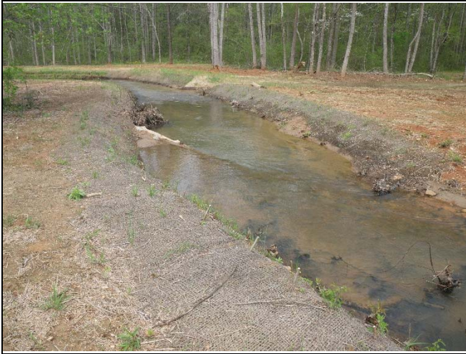
Photo 7. Mainstem Photo Point 4 (PP4) – Station 20+30 (April 17, 2015) downstream from left bank.
