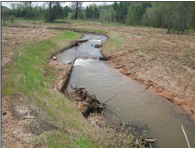
Photo 5. Mainstem Photo Point 3 – Station 24+70 (April 17, 2015) upstream from right bank.
