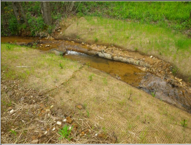
Photo 48. UT3 Photo Point 9 – Station 1+89 (April 17, 2015) upstream to structure.
