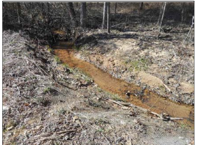
Photo 47. UT3 Photo Point 8 – Station 2+70 (February 2, 2016) upstream to structure.
