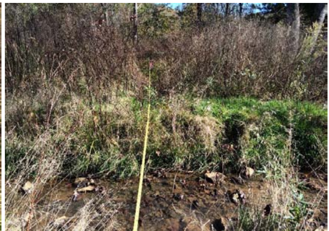
Looking at the Right Bank
