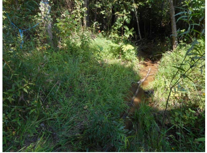
Photo 49. UT3 Photo Point 10 – Station 0+60 (August 30, 2016) downstream to structure.
