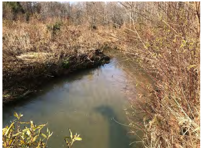
Photo 6. Mainstem Photo Point 3 – Station 24+70 (November 18, 2018) downstream from right bank.
