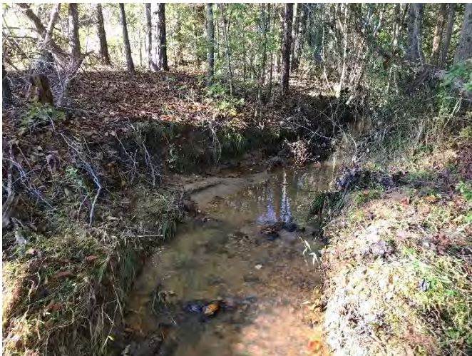
Photo 46. UT3 Photo Point 7 – Station 3+60 (October 18, 2018) upstream to structure.
