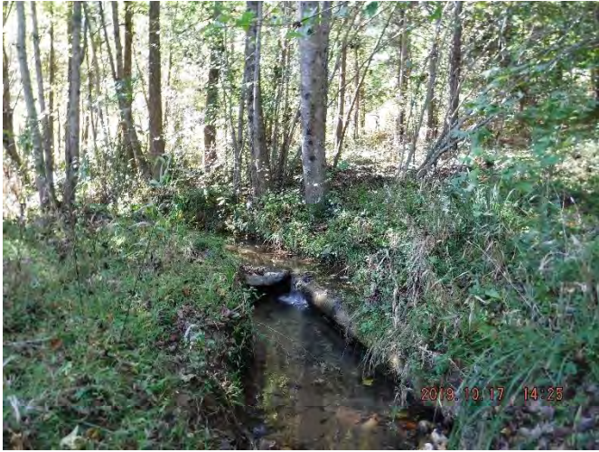
Photo 48. UT3 Photo Point 9 – Station 1+90 (October 17, 2019) upstream to structure.
