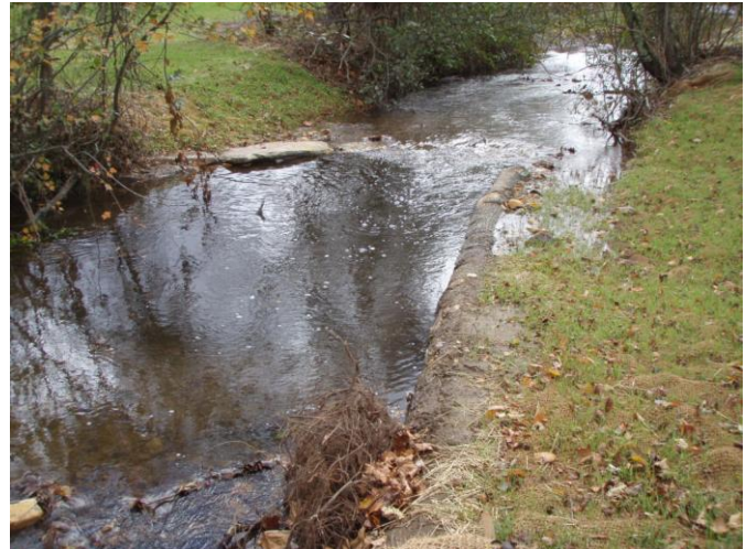
Log vane, root wads, and bank shaping, sta. 4+50, facing upstream, 19 October 2011.
