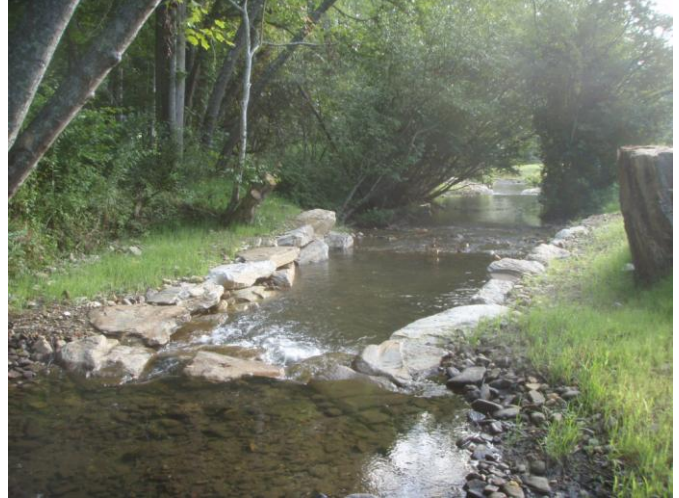
Cross vane, sta. 0+50, facing downstream, 14 August 2011.
