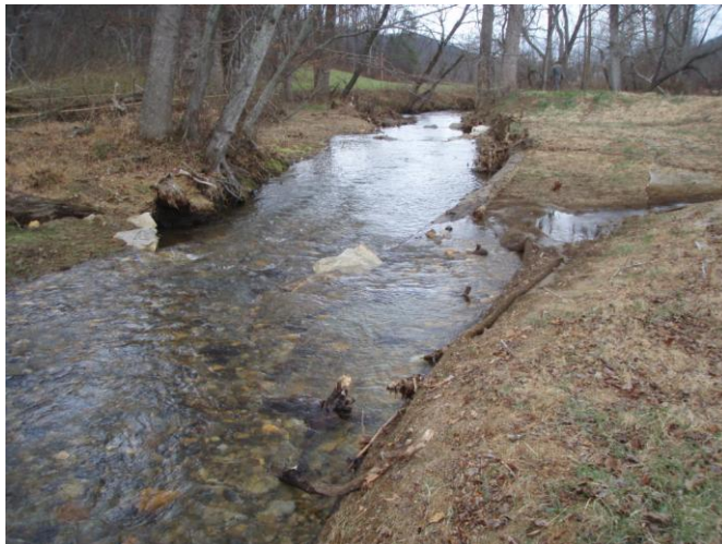
Log vane at sta. 1+00 to 1+50, facing downstream 5 December. 2011.
