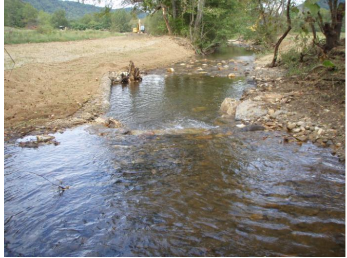
Bank shaping, log vane, and riffle construction, sta. 0+25, 22 September 2011.
