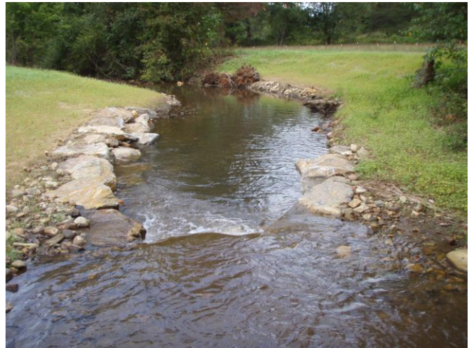
Bank sloping and J-hook, sta. 9+25 to 10+00, 22 September 2011.
