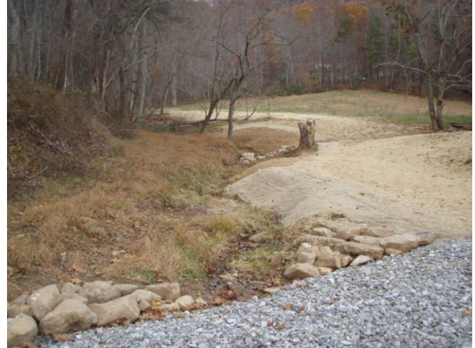
UT3 above ford, invasive removal, cattle exclusion, and bank shaping, facing upstream, 9 November 2011.
