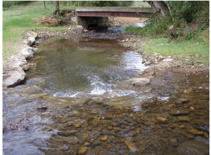
J-hook at sta. 12+75, lower end of Bura/Roberson properties, 22 September 2011.
