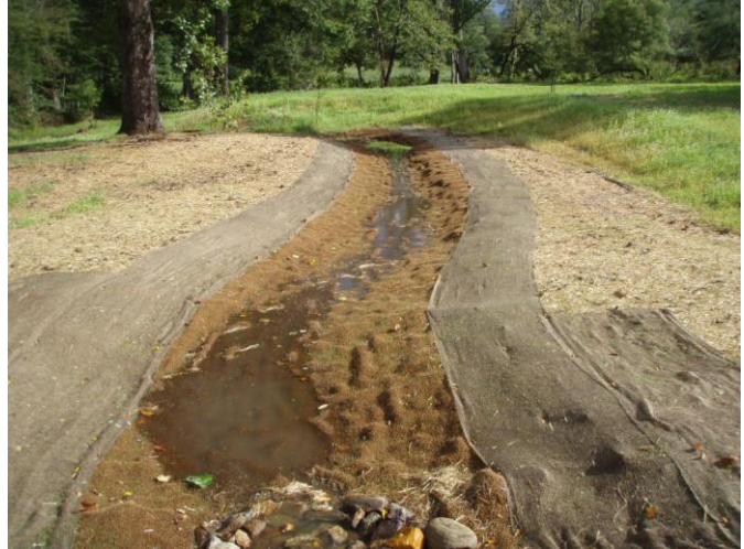
UT2 restored portion, east of Canterfield Lane, 5 December 2011.
