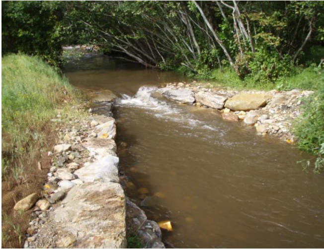
Rock vane after construction, sta. 1+50, facing upstream, 5 September 2011.
