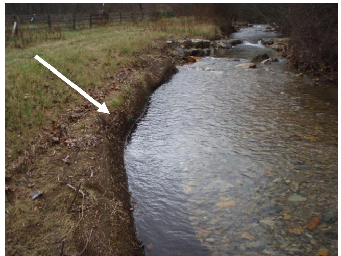
Left channel bank instability after flood damage, sta. 1+75 to 2+25, 5 December 2012.
