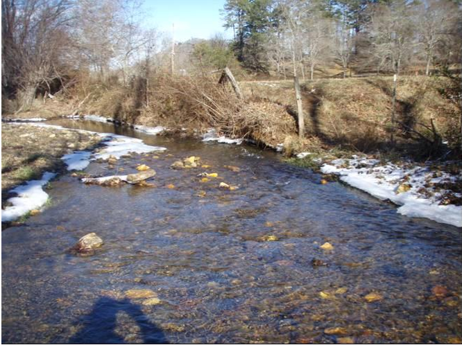
Outside meander bend bank stress, sta. 7+25 to 8+00, facing downstream, 22 January 2009.
