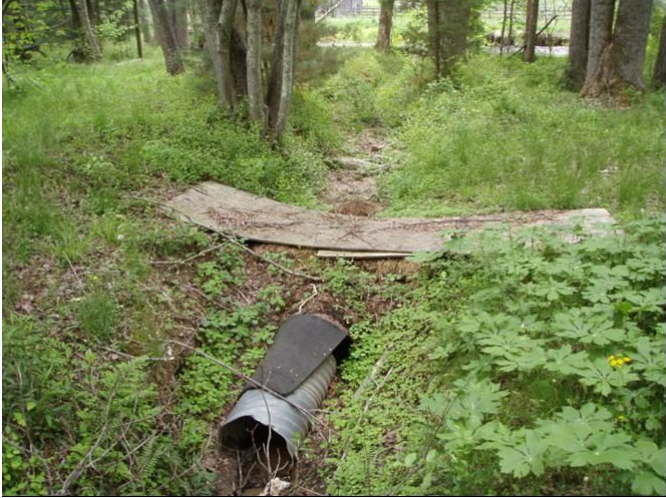
UT1 facing downstream, pre-construction 28 July 2009.
