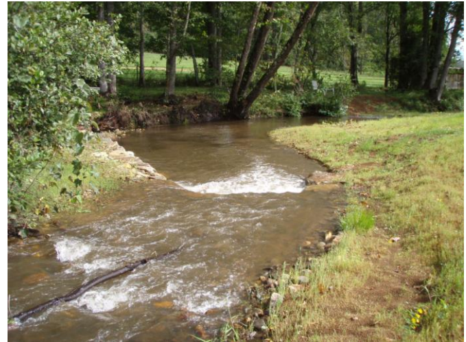
J-hook, sta. 2+50, facing downstream, 5 September 2011.
