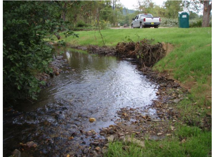
Bank shaping, root wads, and toe-wood, sta. 11+50 to 12+00, 22 September 2011.
