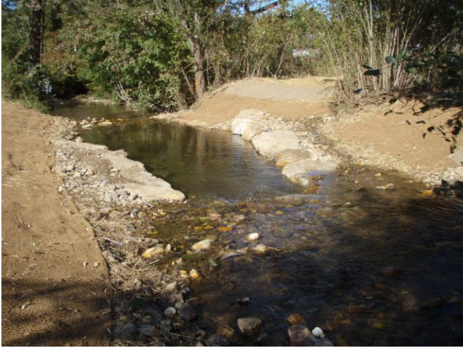
Cross vane, riffle construction, and bank shaping, sta. 6+75, 4 October 2011.
