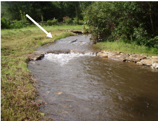
Left channel bank under stable condition, sta. 2+00, facing upstream, 5 September 2011.
