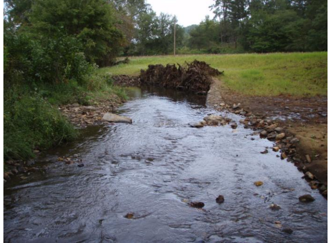
Log vane, root wad, and bank shaping, sta. 7+25 to 8+00, 22 September 2011.
