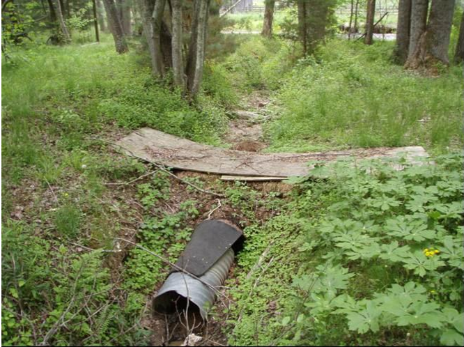
UT1 facing downstream, pre-construction 28 July 2009.
