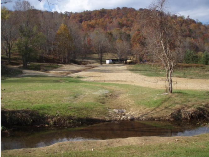
UT3 lower at confluence with SHC, Priority I restoration, facing upstream, 15 November 2011.
