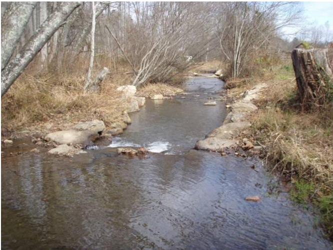
Cross vane, sta. 0+50, facing downstream, 20 November 2012.
