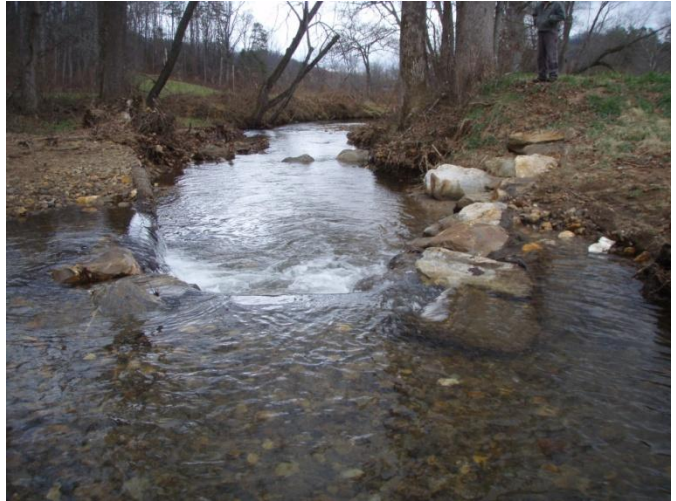
Log vane at sta. 1+50 to 2+50, facing downstream, 5 December 2011.
