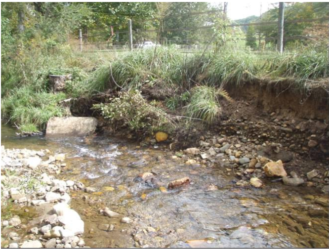
Right bank erosion, sta. 5+50, pre-construction, 30 September 2008.
