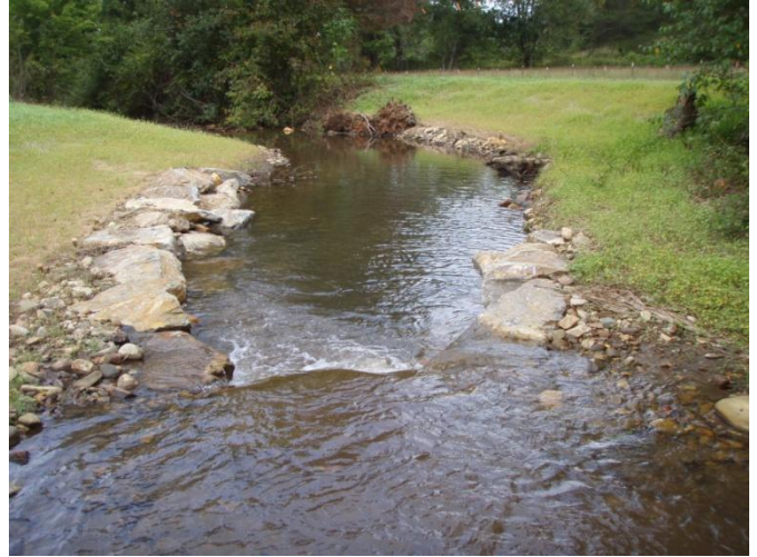
Bank sloping and J-hook, sta. 9+25 to 10+00, 22 September 2011.
