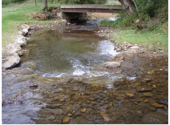
J-hook sta. 12+75, lower end of Bura/Roberson properties, 22 September 2011.
