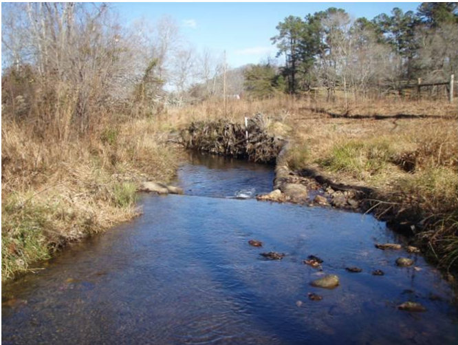
Log vane, root wad, and bank shaping, sta. 7+25 to 8+00, 20 November 2012.
