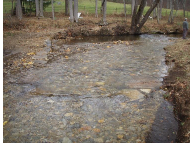
Aggradation and bar formation in meander below J-hook after flood event, sta. 2+50, facing downstream, 5 December 2011.
