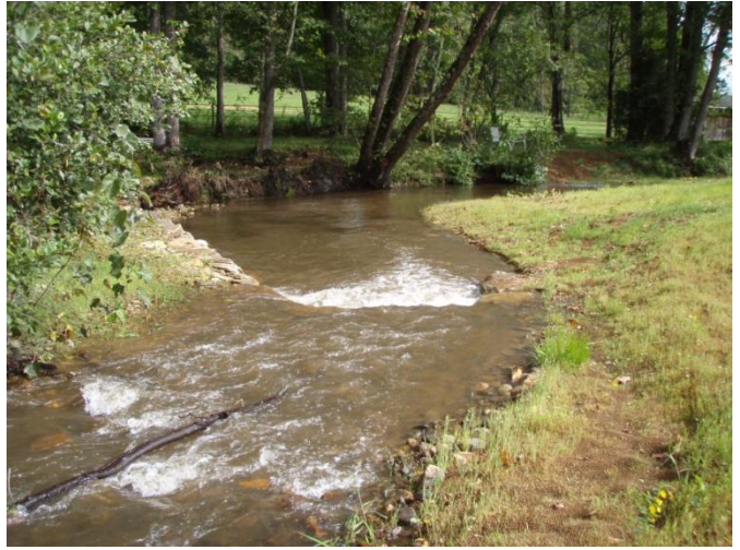
J-hook, sta. 2+50, facing downstream, 5 September 2011.
