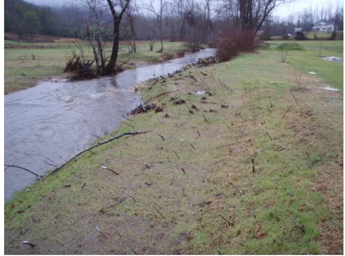
Log vane, root wads, and bank shaping, sta. 2+25 to 3+50, facing downstream, 7 December 2011.
