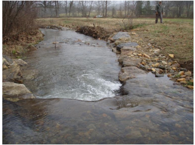
J-hook, sta. 5+00, facing downstream, 5 December 2011.
