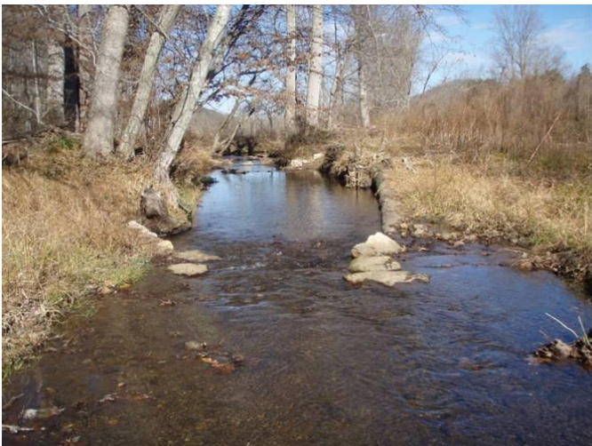
Log vane sta. 1+00 to 1+50, facing downstream, 20 November 2012.
