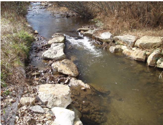
Rock vane, sta. 1+50, facing upstream, 20 November 2012.
