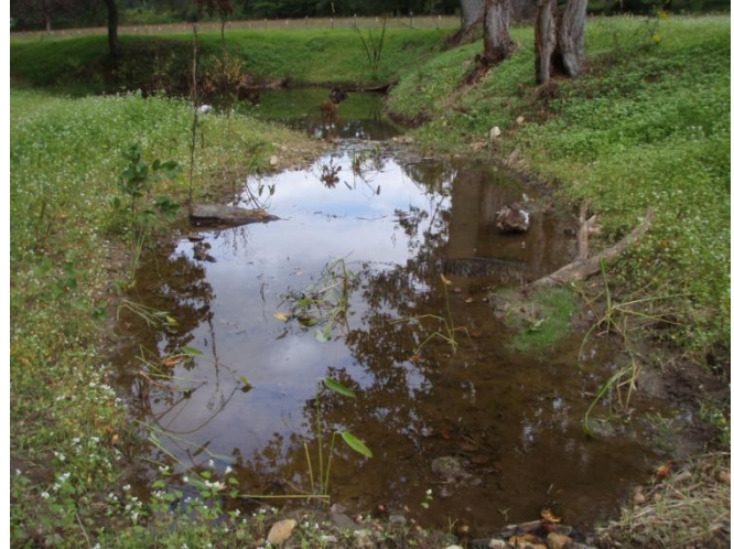
Enhancement to Wetland D, facing downstream, 22 September 2011.
