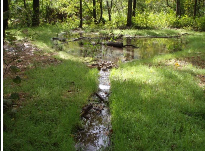
UT1 Priority I channel construction, above vernal pond, 5 September 2011.
