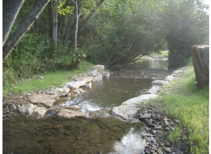
Cross vane, sta. 0+50, facing downstream, 14 August 2011.
