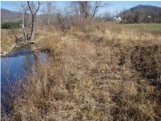
Log vane, root wads, and bank shaping, sta. 2+25 to 3+50, facing Downstream, 20 November 2012.
