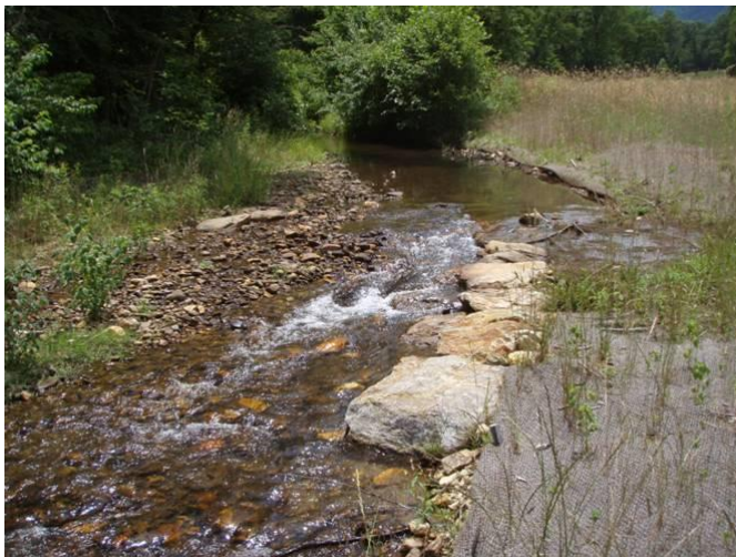
Aggradation and bar formation below J-hook, sta. 9+25 to 9+50, facing upstream, 14 June 2012
