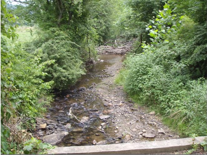
J-hook proposed, sta. 0+50, facing downstream, 25 July 2008, pre-construction.
