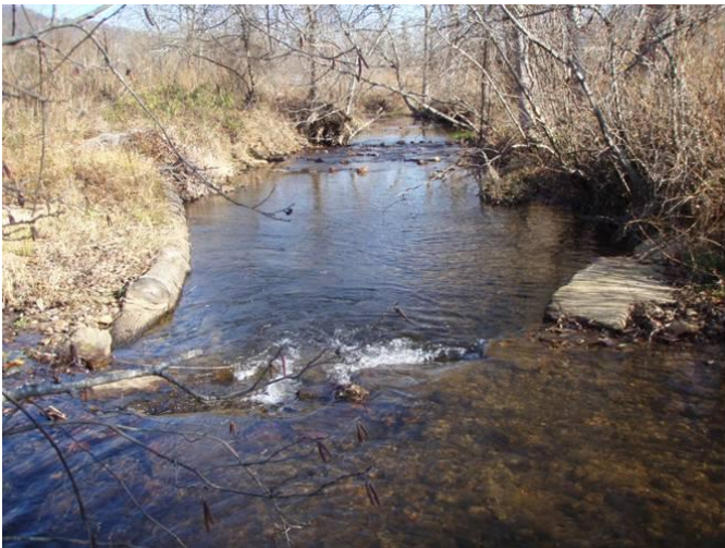
Log vane, root wads, and bank shaping, sta. 4+50, facing downstream 20 November 2012.
