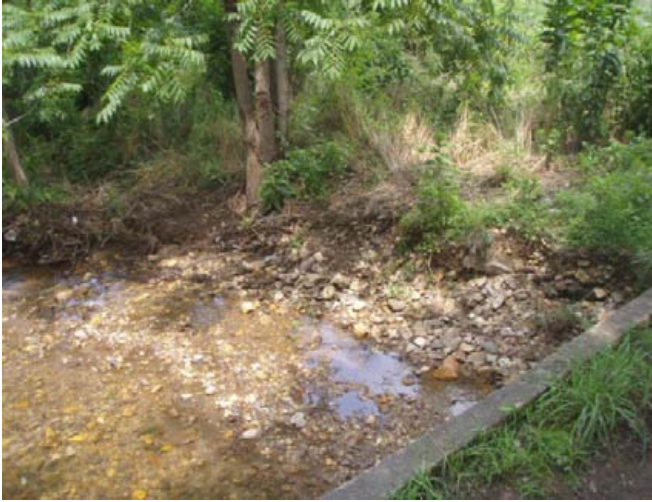
Right bank scour during 5 May 2013 flood event, sta. 0+00 to 0+20, facing downstream, 18 July 2013.
