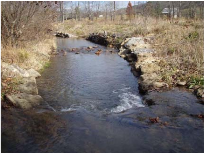
J-hook, sta. 5+00, facing downstream, 20 November 2012.
