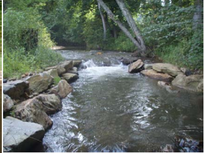
Cross vane after 5 May 2013 flood event, facing upstream, sta. 0+50, 18 July 2013.
