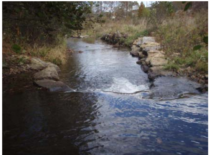
J-hook, sta. 5+00, facing downstream, 29 October 2013.
