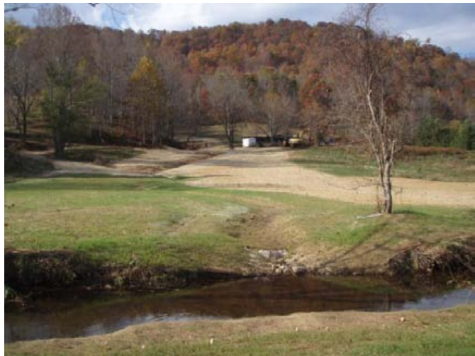
UT3 lower at confluence with SHC, Priority I restoration, facing upstream, 15 November 2011.
