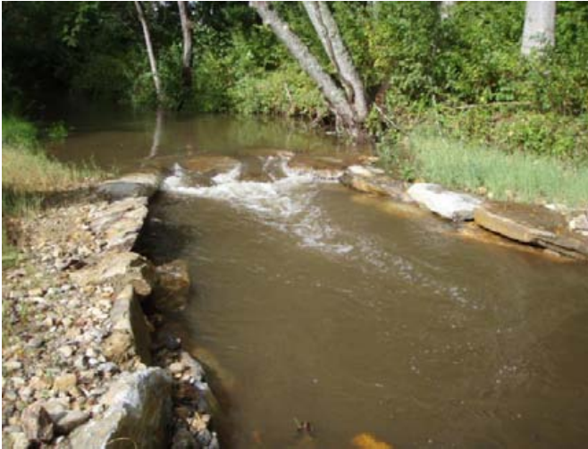
Cross vane after construction, facing upstream, sta. 0+50 14 Aug 2011.
