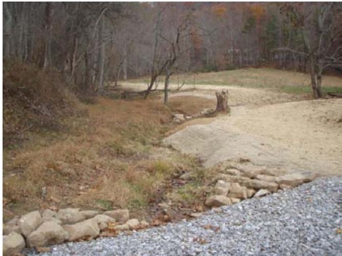
UT3 above ford, invasive removal, cattle exclusion, and bank shaping, facing upstream, 9 November 2011.
