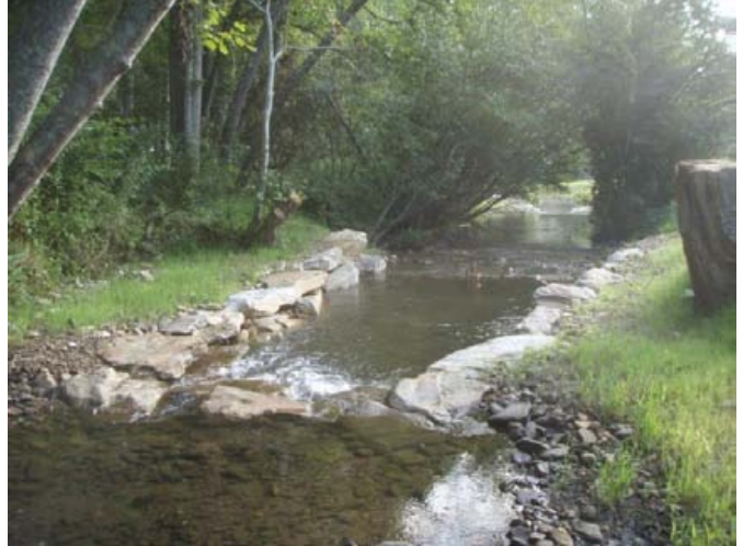
Cross vane, sta. 0+50, facing downstream, 14 August 2011.
