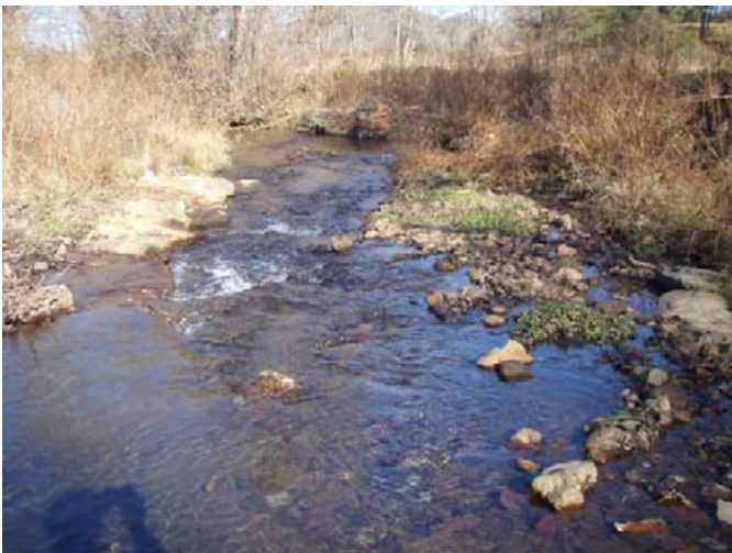
Bank sloping and J-hook, sta. 9+25 to 10+00, 14 June 2012.
