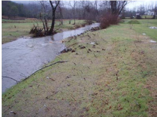
Log vane, root wads, and bank shaping, sta. 2+25 to 3+50, facing downstream, 7 December 2011.
