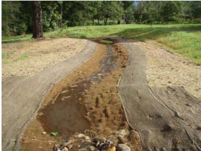
UT2 restored portion, east of Canterfield Lane, 5 September 2011.
