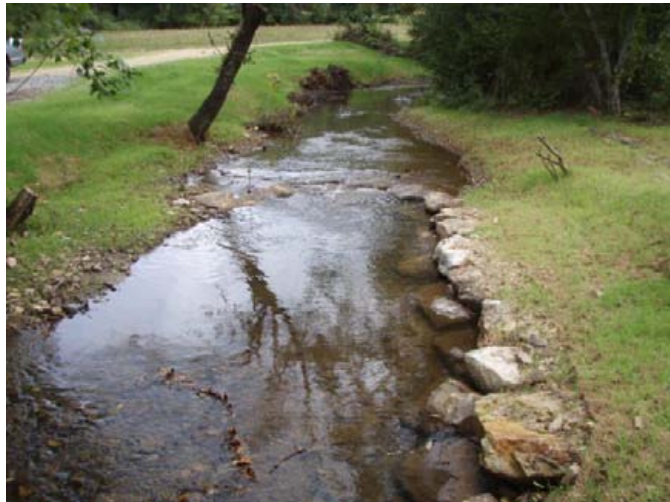
J-hook, sta. 12+75, after construction, facing upstream, 22 Sept 2011.
