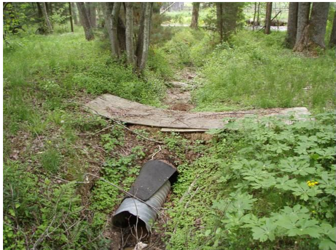
UT1 facing downstream, pre-construction 28 July 2009.
