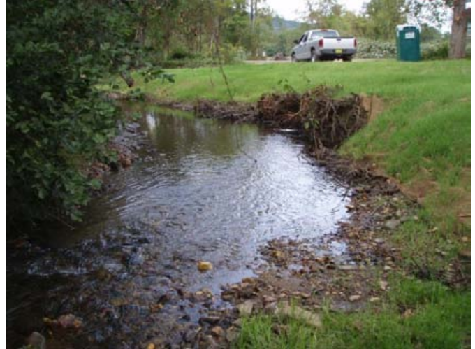
Bank shaping, root wads, and toe-wood, sta. 11+50 to 12+00, facing downstream, 22 September 2011.
