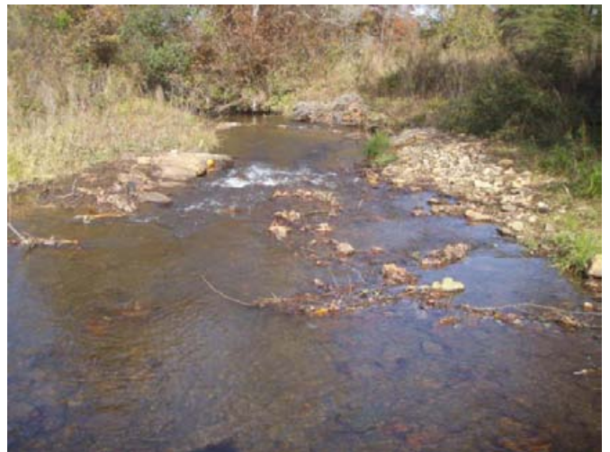
Bank sloping and J-hook, sta. 9+25 to 10+00, 29 October 2013.
