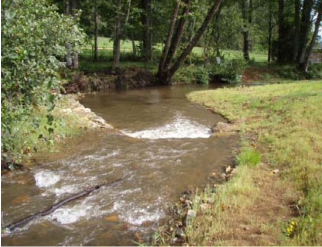
J-hook and meander post construction, sta. 2+50, facing downstream, 5 September 2011.
