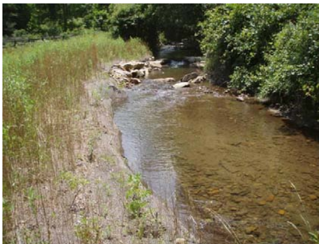
Right channel bank instability after flood, sta. 1+75 to 2+25, facing upstream, 14 June 2012.
