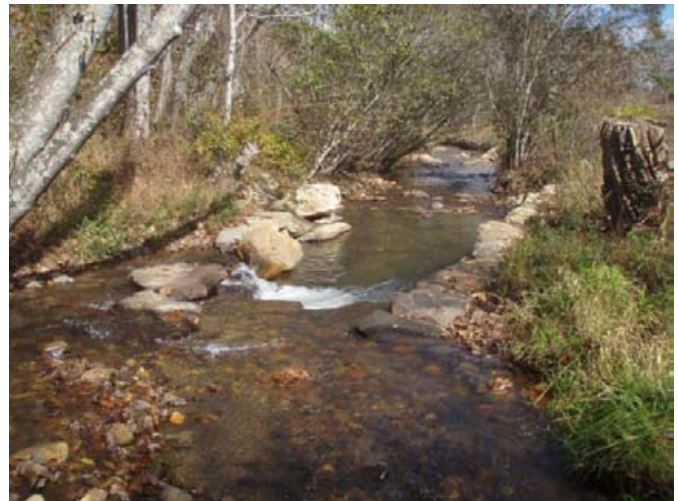
Cross vane, sta. 0+50, facing downstream, 29 October 2013.
