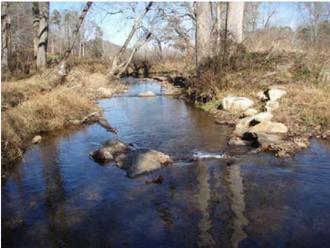
Log vane sta. 1+50 to 2+50, facing downstream, 20 November 2012.
