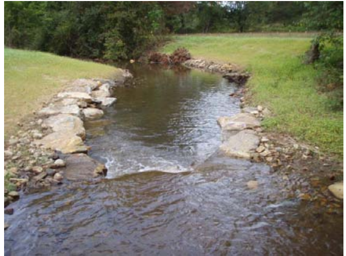
Bank sloping and J-hook, sta. 9+25 to 10+00, 22 September 2011.
