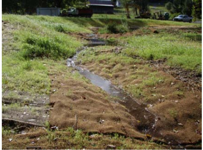
Lower portion of UT2 at confluence with SHC, facing upstream, 5 September 2011.
