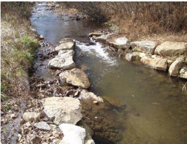
Rock vane, sta. 1+50, facing upstream, 20 November 2012.
