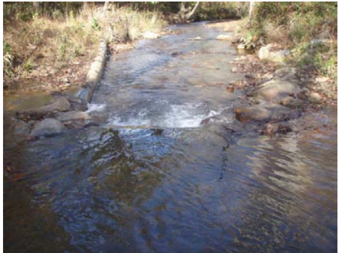
Log vane sta. 1+50 to 2+50, facing downstream, 29 October 2013.
