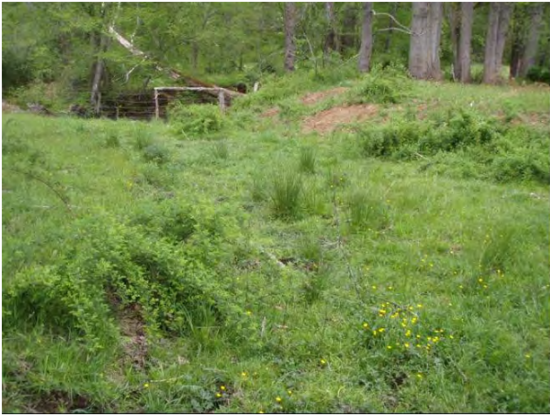
Lower portion of UT2 abandoned channel at confluence with SHC, Pre-construction, facing downstream, 26 April 2010.
