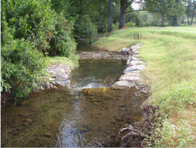
J-hook vane after construction, sta. 5+75, facing downstream, 14 August 2011.
