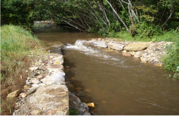
Rock vane after construction, sta. 1+50, facing upstream, 5 September 2011.
