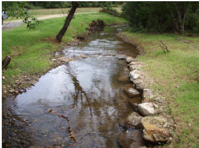
J-hook, sta. 12+75, after construction, facing upstream, 22 Sept 2011.
