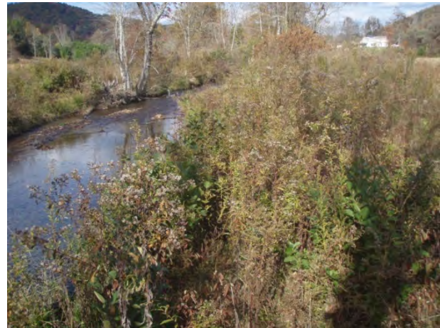
Log vane, root wads, and bank shaping, sta. 2+25 to 3+50, facing downstream, 29 October 2013.
