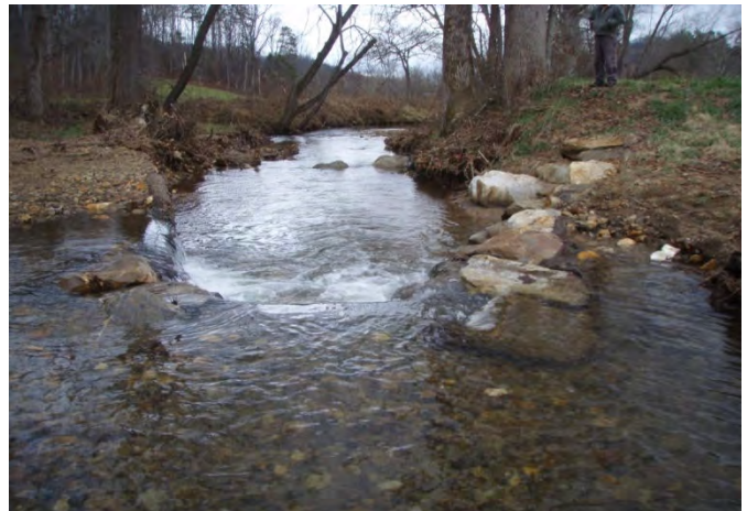
Log vane at sta. 1+50 to 2+50, facing downstream, 5 December 2011.
