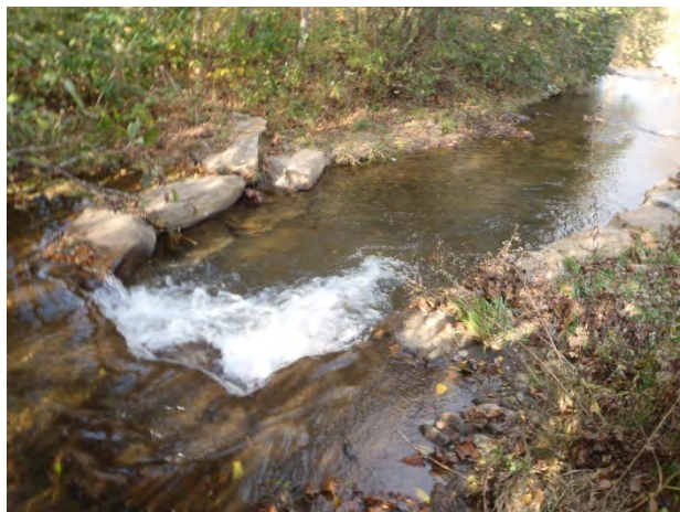
J-hook, sta. 5+00, facing downstream, 12 November 2014.
