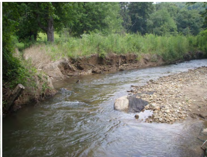
Right bank scour and erosion during 5 May 2013 flood event, facing upstream, sta. 12+50, 18 July 2013.
