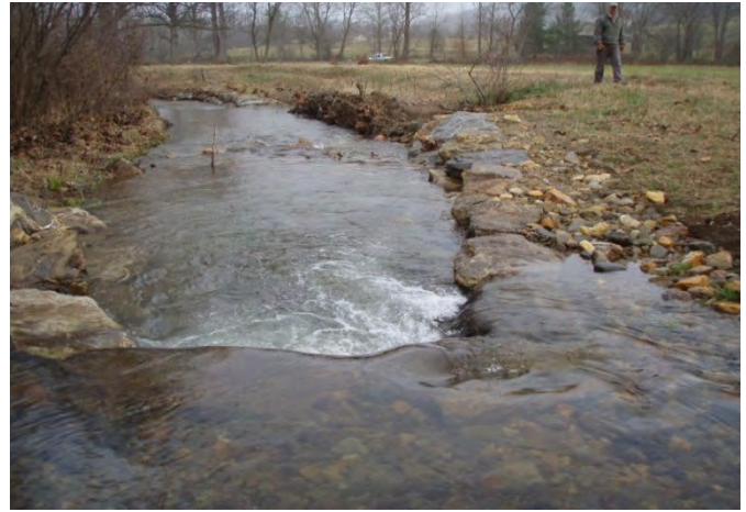
J-hook, sta. 5+00, facing downstream, 5 December 2011.
