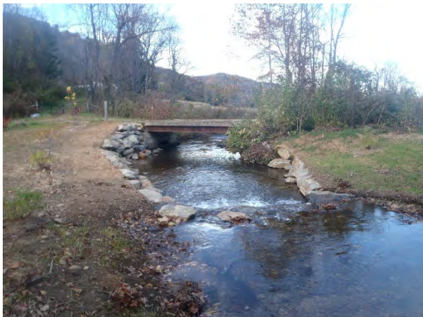
J-hook sta. 12+75, lower end of Bura/Roberson properties, 12 Nov 2014.
