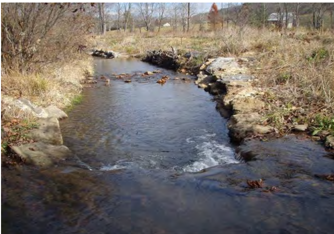
J-hook, sta. 5+00, facing downstream, 20 November 2012.
