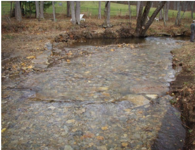
Aggradation and bar formation in meander below J-hook after flood event, sta. 2+50, facing downstream, 5 December 2011.
