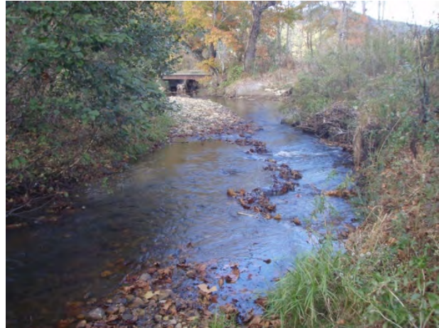
Bank shaping, root wads, and toe-wood, sta. 11+50 to 12+00, facing downstream, 20 November 2012.
