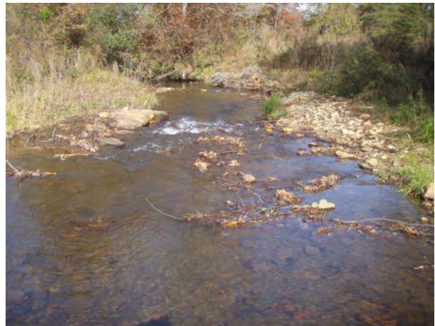
Bank sloping and J-hook, sta. 9+25 to 10+00, 29 October 2013.
