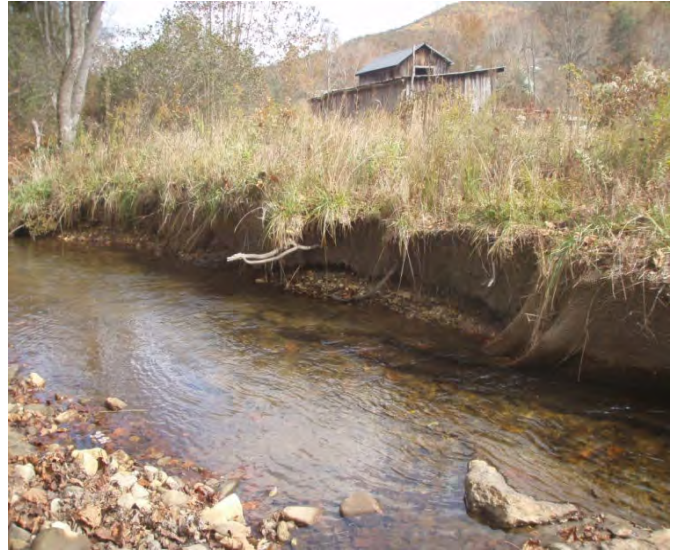
Right channel bank condition after 5 May 2013 flood, sta. 1+75 to 2+25, facing downstream, 29 October 2013.
