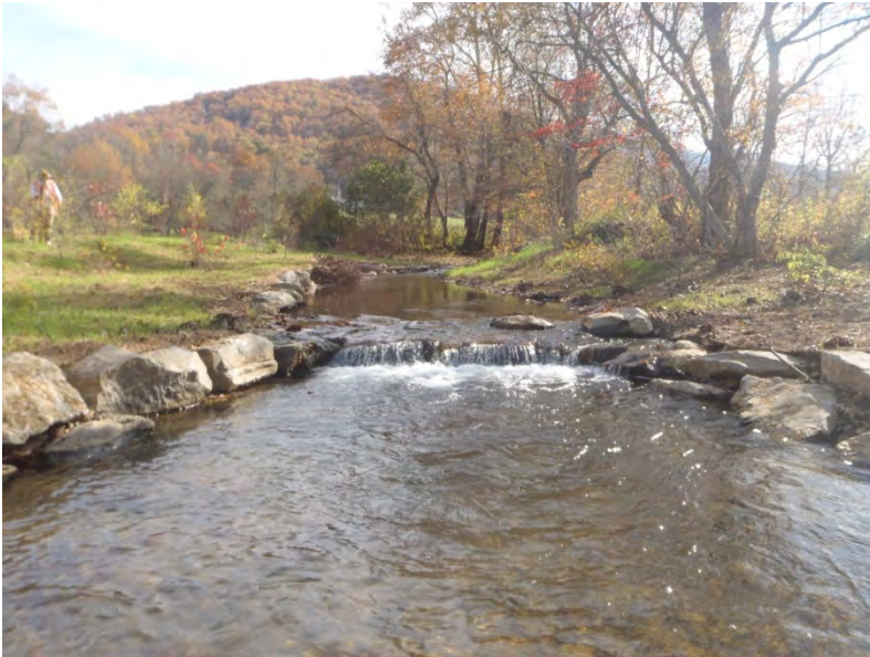
PA-7 station 12+75 facing upstream was repaired and is no longer considered a problem 28 October 2014
