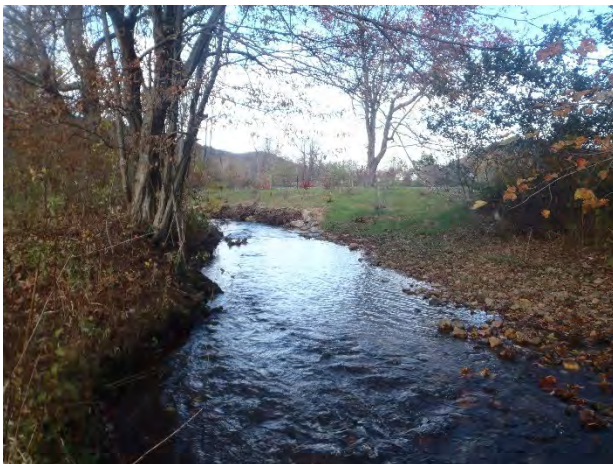
Bank shaping, root wads, and toe-wood, sta. 11+50 to 12+00, facing downstream, 12 Nov 2014.
