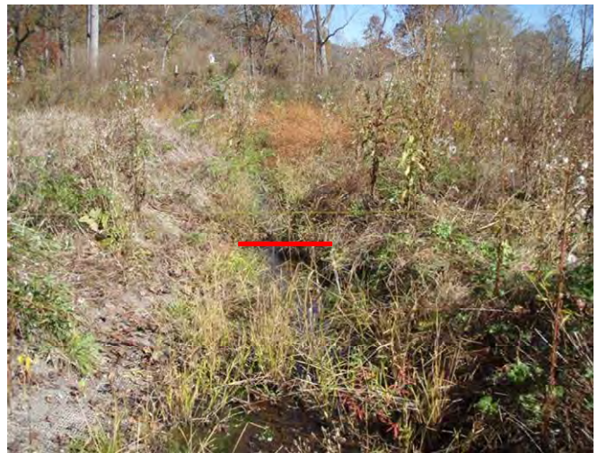
Cross-section 1, UT2 facing downstream, 24 October 2012, MY1.
