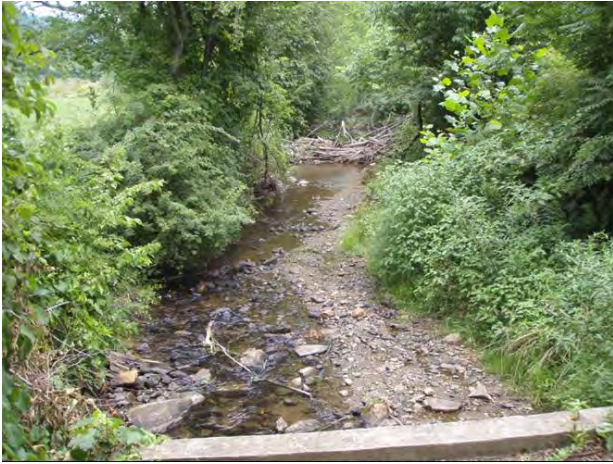
J-hook proposed, sta. 0+50, facing downstream, 25 July 2008, pre-construction.
