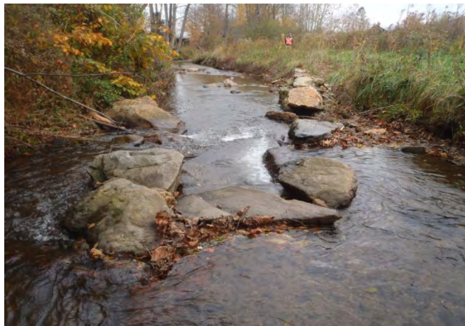
Rock vane, sta 1+50 facing downstream 28, October 2014
