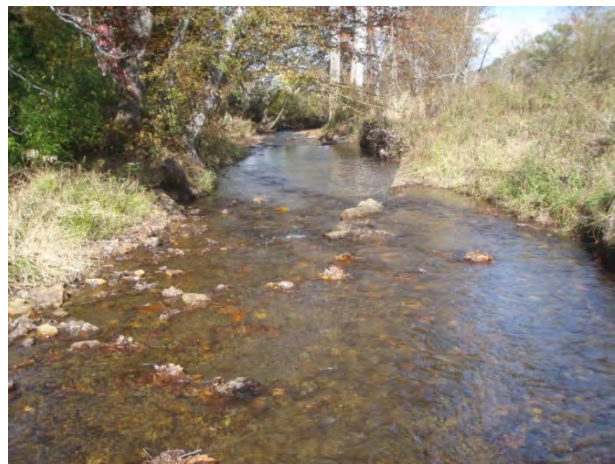
Log vane sta. 1+00 to 1+50, facing downstream, 29 October 2013.
