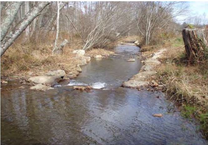
Cross vane, sta. 0+50, facing downstream, 20 November 2012.
