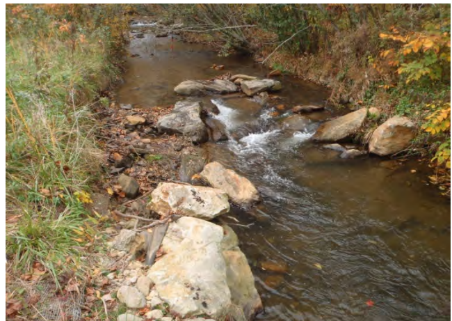
Rock vane, sta 1+50 facing upstream, 28, October 2014
