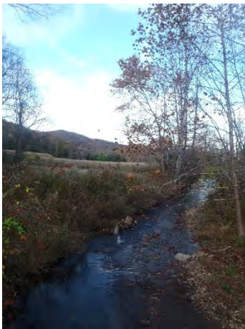
Bank shaping, log vane, and riffle construction, sta. 0+25, 12 Nov 2014.
