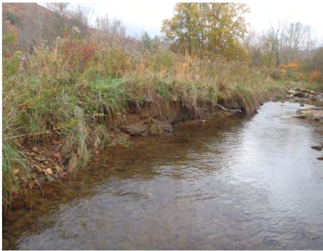
Right channel bank condition sta. 1+75 to 2+25 facing upstream, 20 October 2014.
