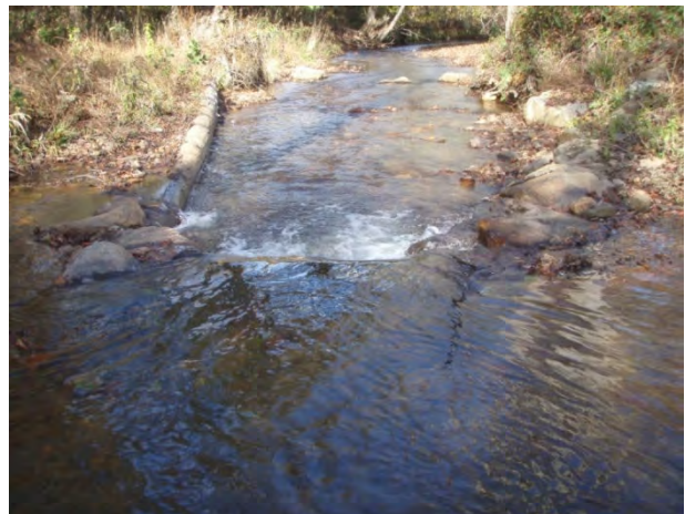
Log vane sta. 1+50 to 2+50, facing downstream, 29 October 2013.
