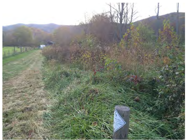
Sta. 6+50 to 8+00, right bank facing upstream, 12 Nov 2014.
