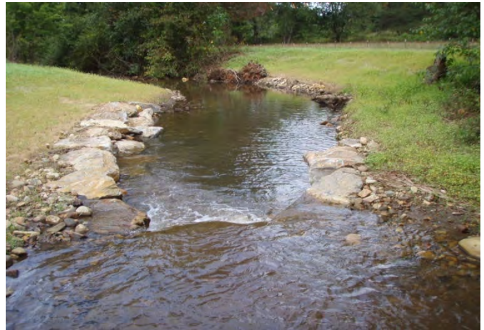
Bank sloping and J-hook, sta. 9+25 to 10+00, 22 September 2011.
