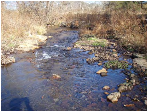
Bank sloping and J-hook, sta. 9+25 to 10+00, 14 June 2012.
