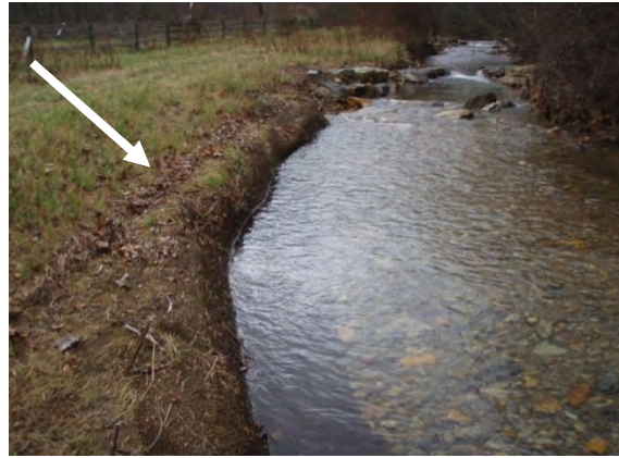
Right channel bank instability after flood damage, sta. 1+75 to 2+25, facing upstream, 5 December 2011.
