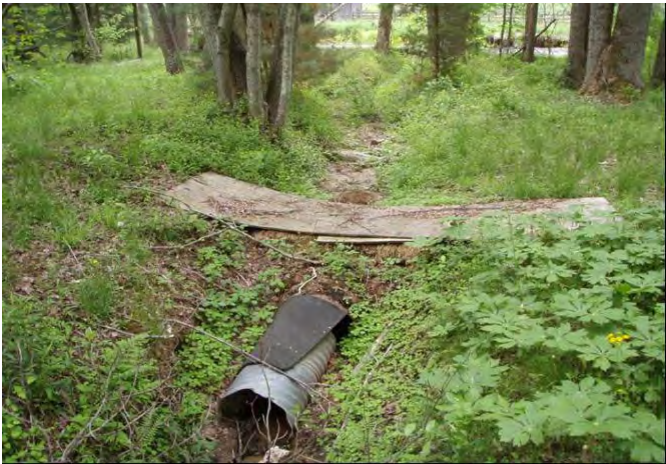
UT1 facing downstream, pre-construction 28 July 2009.
