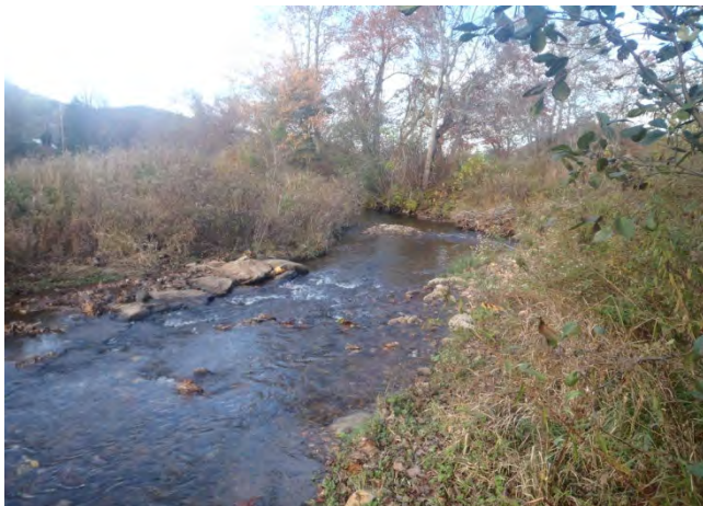
Bank sloping and J-hook, sta. 9+25 to 10+00, 12 Nov 2014.
