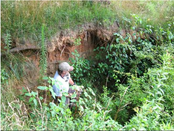
UT3 below ford, severe entrenchment and head cutting, 25 July 2008.
