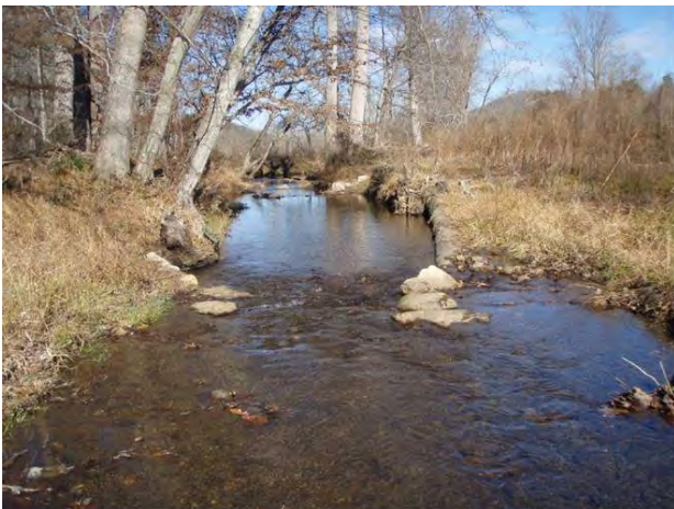
Log vane sta. 1+00 to 1+50, facing downstream, 20 November 2012.
